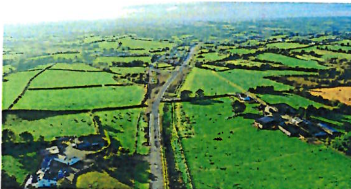
Aerial view southward of the realigned Mainline at the northern tie-in in the townlands of Drumhawragh & Ballytrust.
