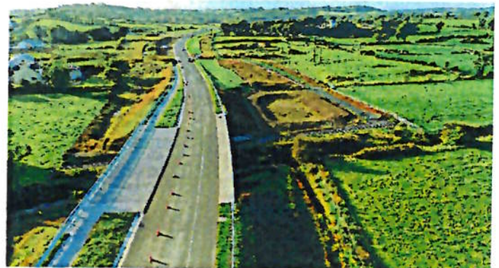
Aerial view south of the new N55 Mainline in the vicinity of Bridge 1 in the townland of Killydoon.
