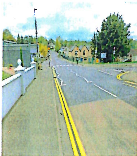
Above: Completed EWS Works N55 Ballinagh
