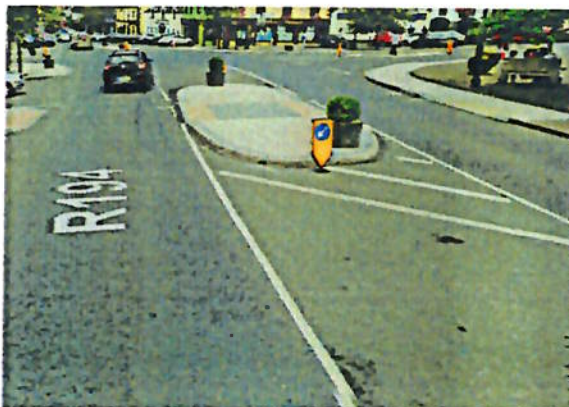
Above: L3503 Carrickallen – Improved Road Surface, Road Markings, High Friction Surfacing and Signage
