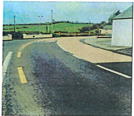
Above: L3503 Carrickallen – Improved Road Surface, Road Markings, High Friction Surfacing and Signage
