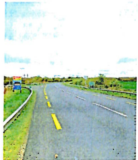
Above: Completed EWS Works N55 Pottahee
