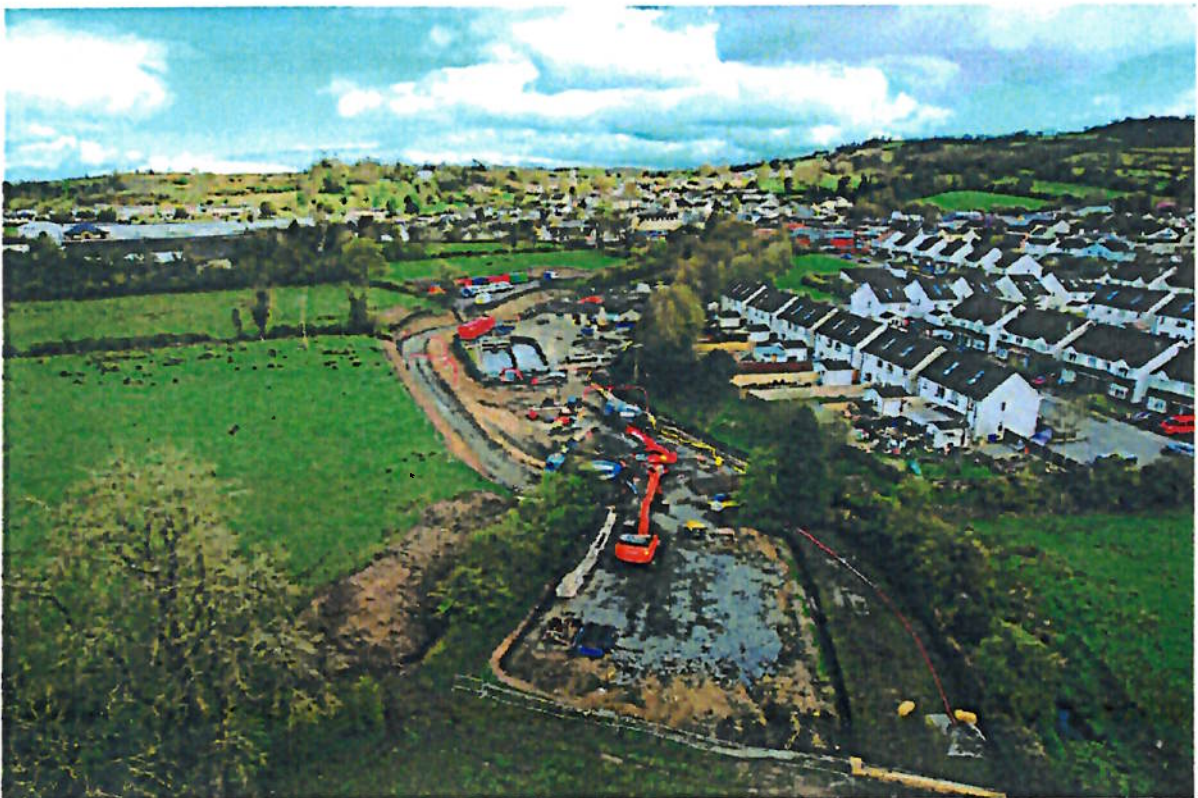
Progress to date on site Upgraded Ballyjamesduff Wastewater Treatment Plant
