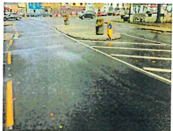
Above: L3503 Carrickallen – Improved Road Surface, Road Markings, High Friction Surfacing and Signage
