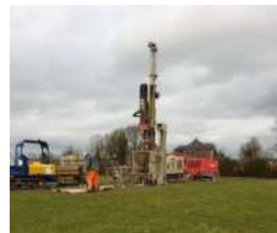
Site investigation - Rotary Coring
