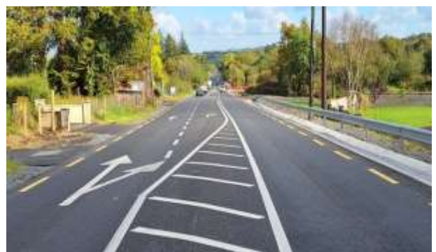
Above : New right turning lanes for southbound traffic turning into the L2508 Caughoo and northbound traffic turning into the L6568 Kilmainham.
