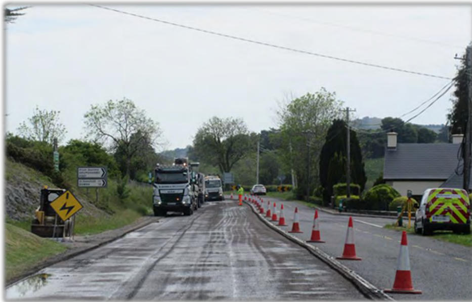
Above: Resurfacing works on the N16 Blacklion West Scheme June 2020
