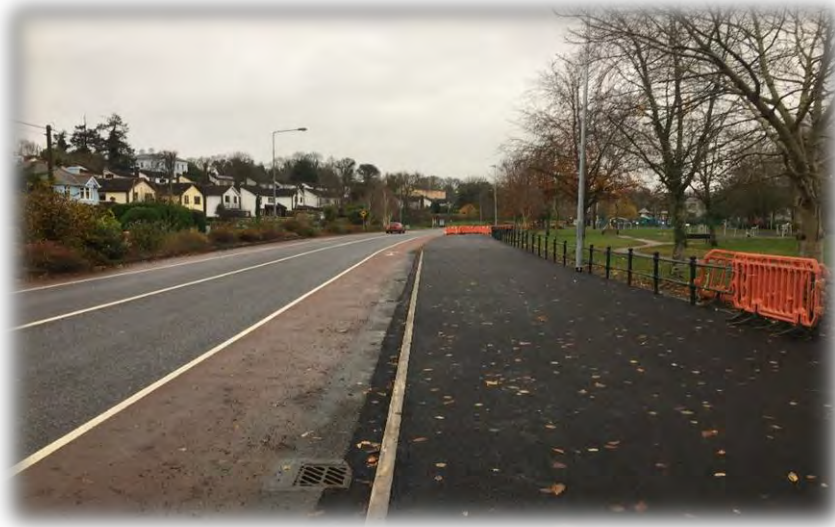
Above: Completed Active Travel Works on the Cathedral Road, Cavan Town
