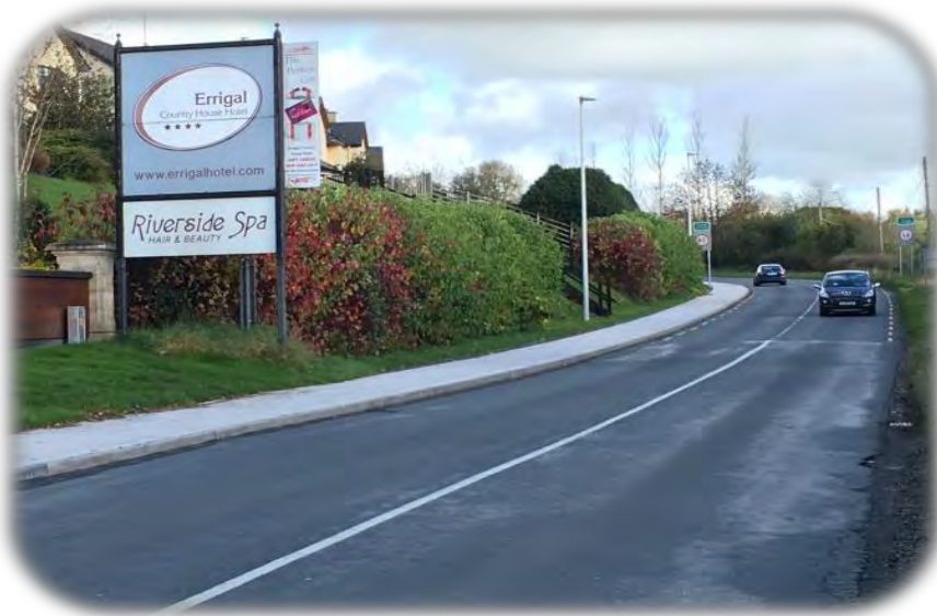
Above: Footpath & Public Lighting on R188 approach to Cootehill
