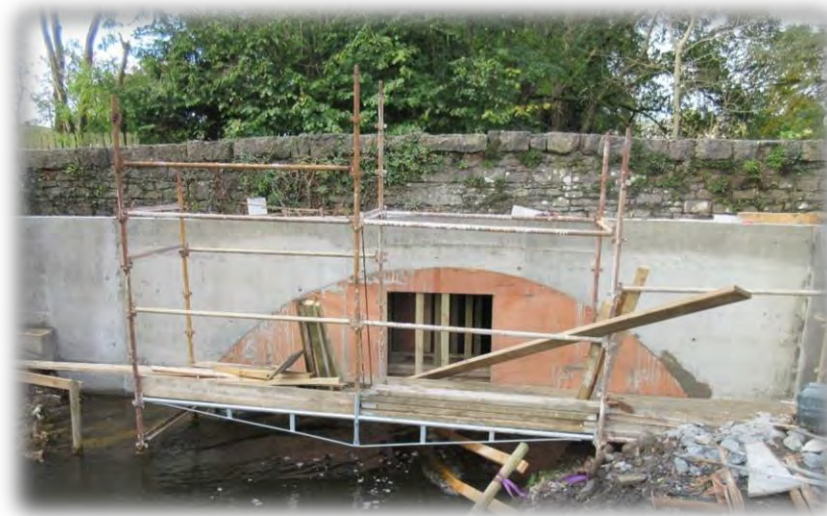
Above: Widening of Drumlark Bridge to accommodate new footpath
