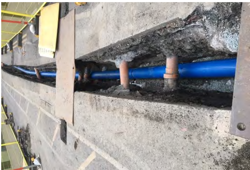
250mm pipe in trench threading under numerous Utility services
