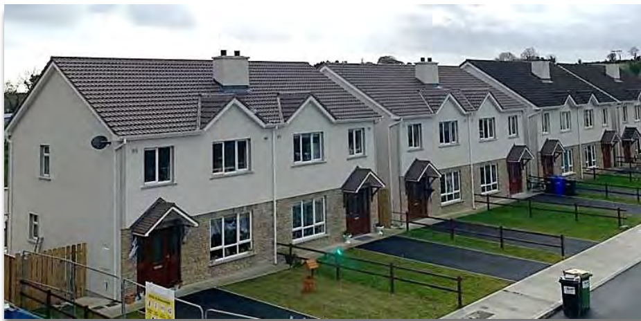
New Housing at Ashgrove, Ballyjamesduff
