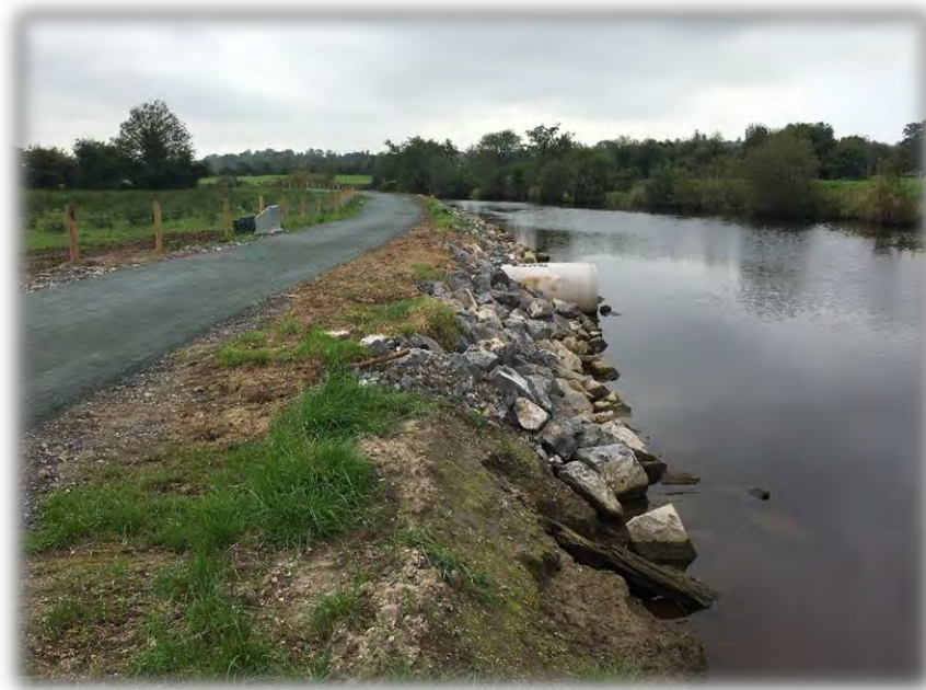
Above: Completed section of the Ballyconnell to Bellaheady recreational trail
