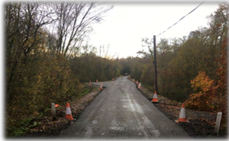
Above: Completed Climate Adaptation Works on the L55321 Drumard/Kilmore
