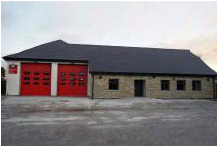
The new Virginia Fire Station which became operational during 2019
