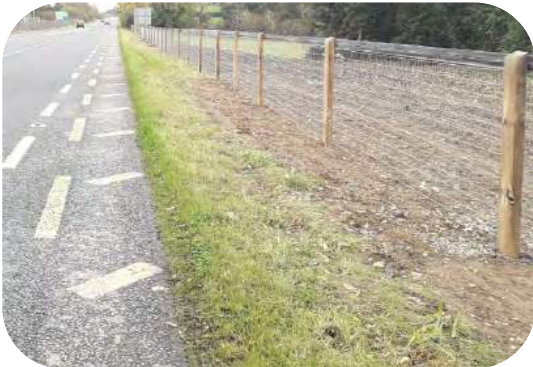
Section of Retro-fit fencing scheme on the N3 at New Inns
