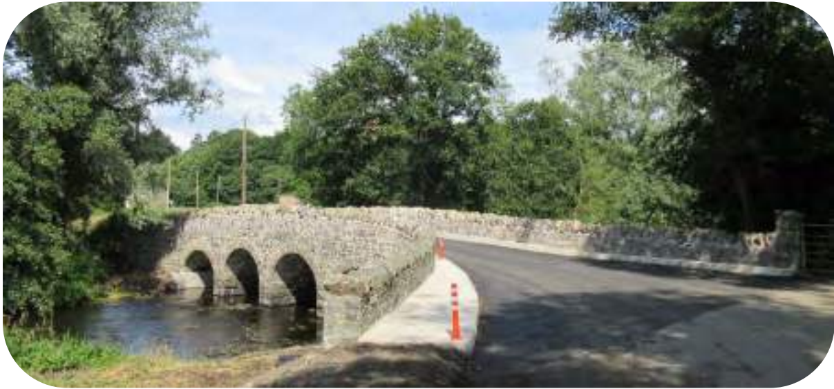
Lisnagoon Bridge – After
