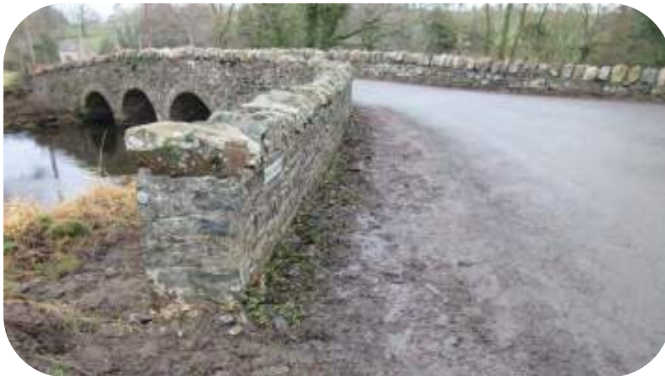
Lisnagoon Bridge - Before
