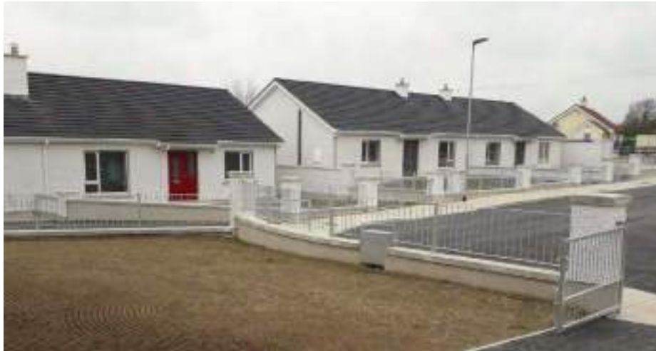
New Housing Scheme at Rosehill, Mullagh completed in 2019.
