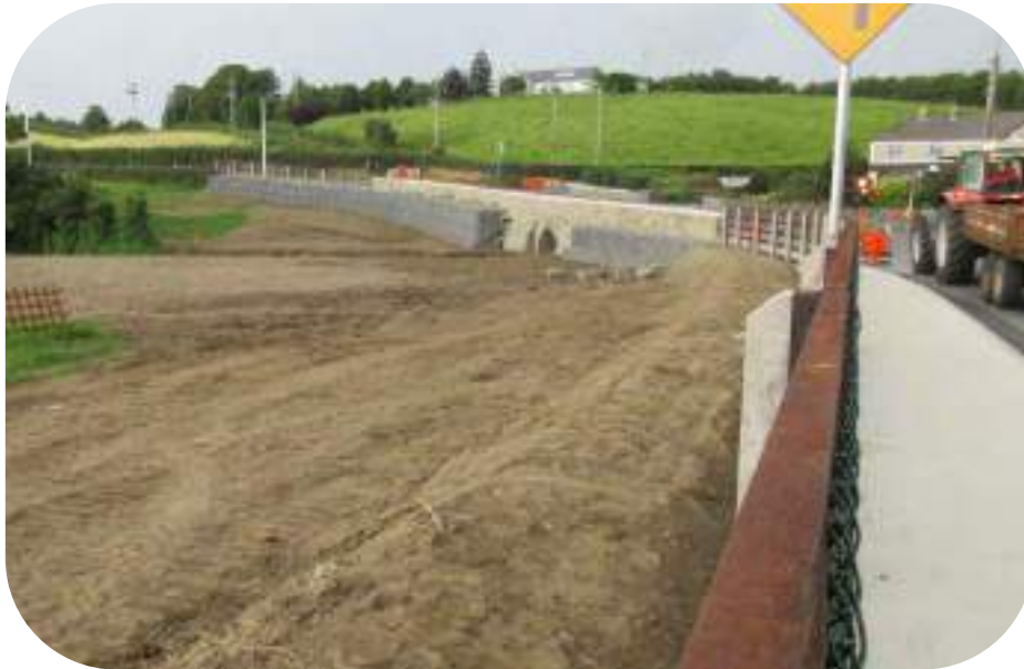
Shercock Bridge – After
