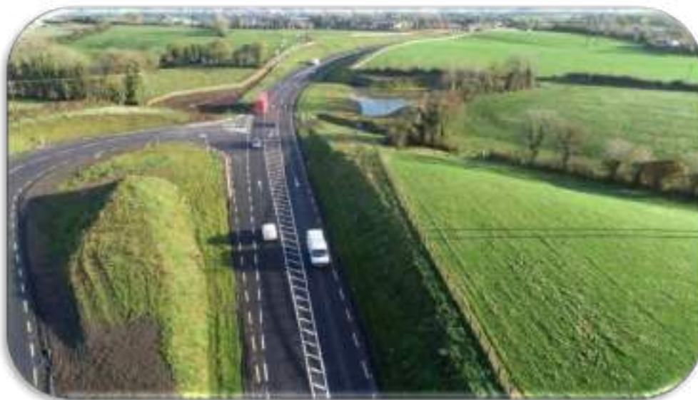
Above: An aerial view of the realigned N55 at Garrymore, and the new junction with the L-6552, complete with dedicated right turning lane.
