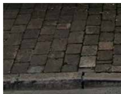
04 Pavement at Henry Street
