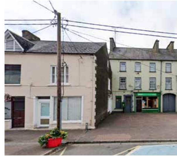
03 Baillieborough Main Street - Existing pole and cables
