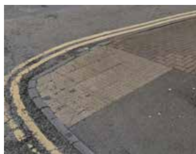
03 Pavement at Thomas Street
