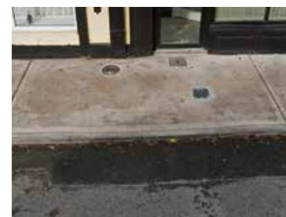
02 Pavement at Barrack Street
