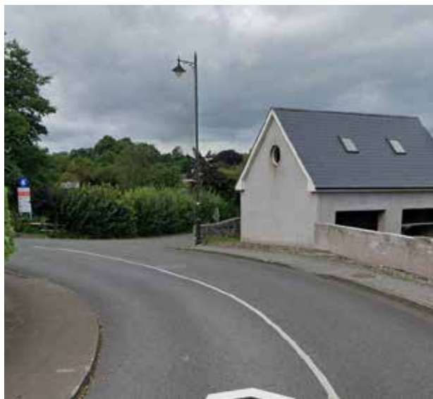
View of roadside
