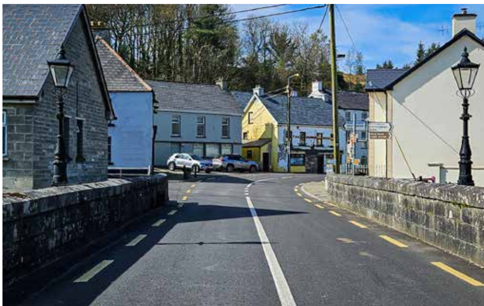
Fig. 10: View from Dowra Bridge towards Main Street.
