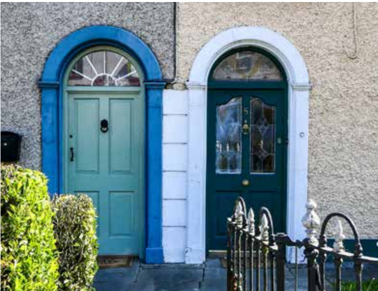
Fig. 19: Examples of tooled stone doorcases found at the northern end of Main Street.
