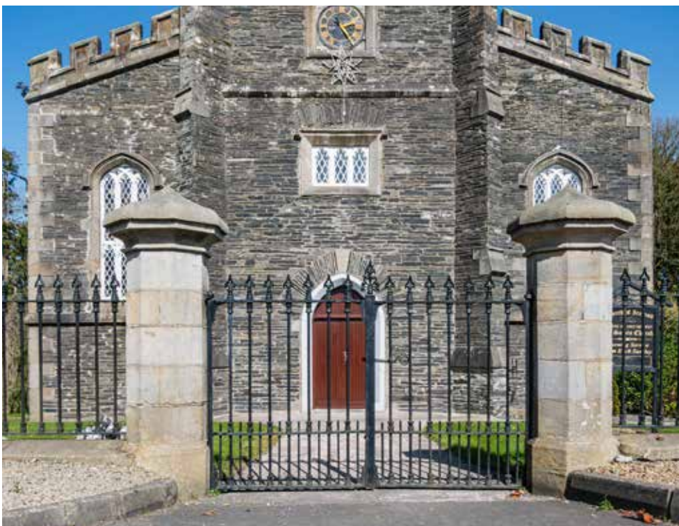
Fig. 17: Sandstone gate piers, gates, and railings at All Saints church.
