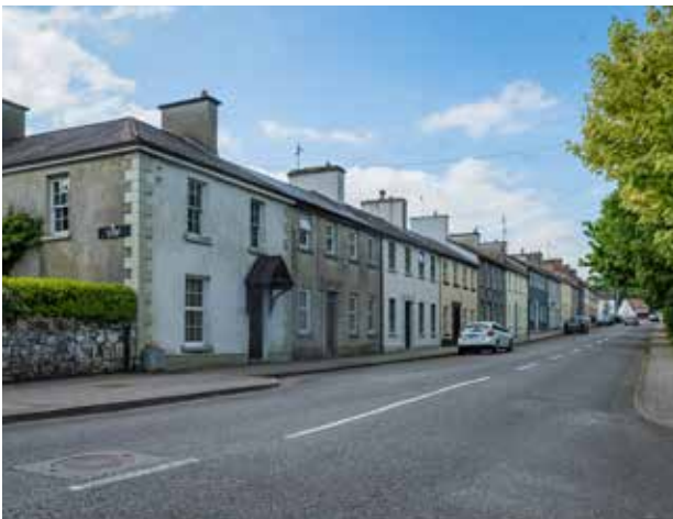
Fig. 9: The Lawn taken from south-western end of street.
