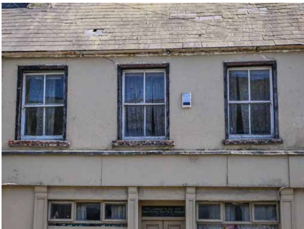
Fig. 21: Timber sash windows on Main Street.
