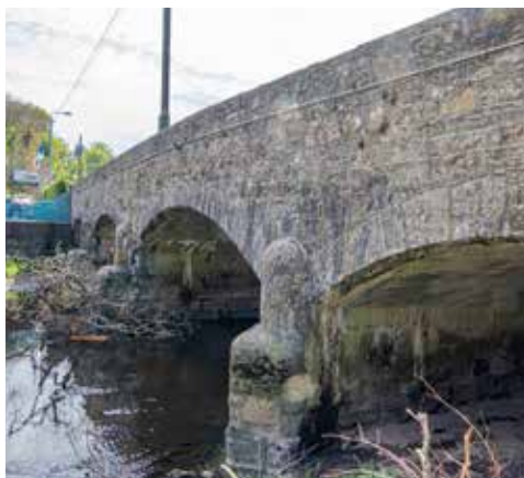
Fig. 16: View of the bridge in Butlersbridge from various aspects.
