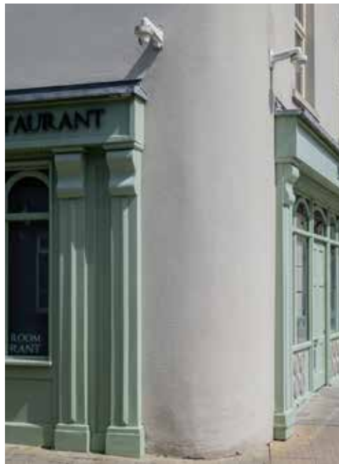
Fig. 15: Curved corners on buildings at the crossroads where Abbey Street crossed Bridge Street.
