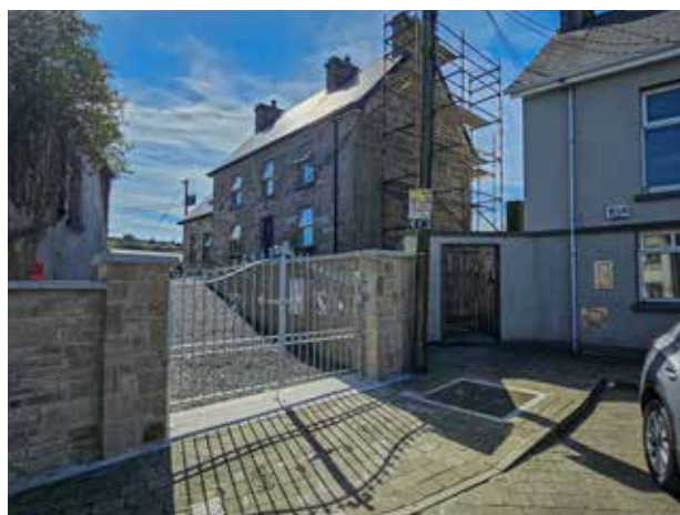
Fig. 18: Stone building at the end of the Main Street, recently restored.
