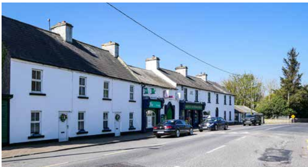
Fig. 10: View of Main Street Mountnugent northwards towards the bridge.
