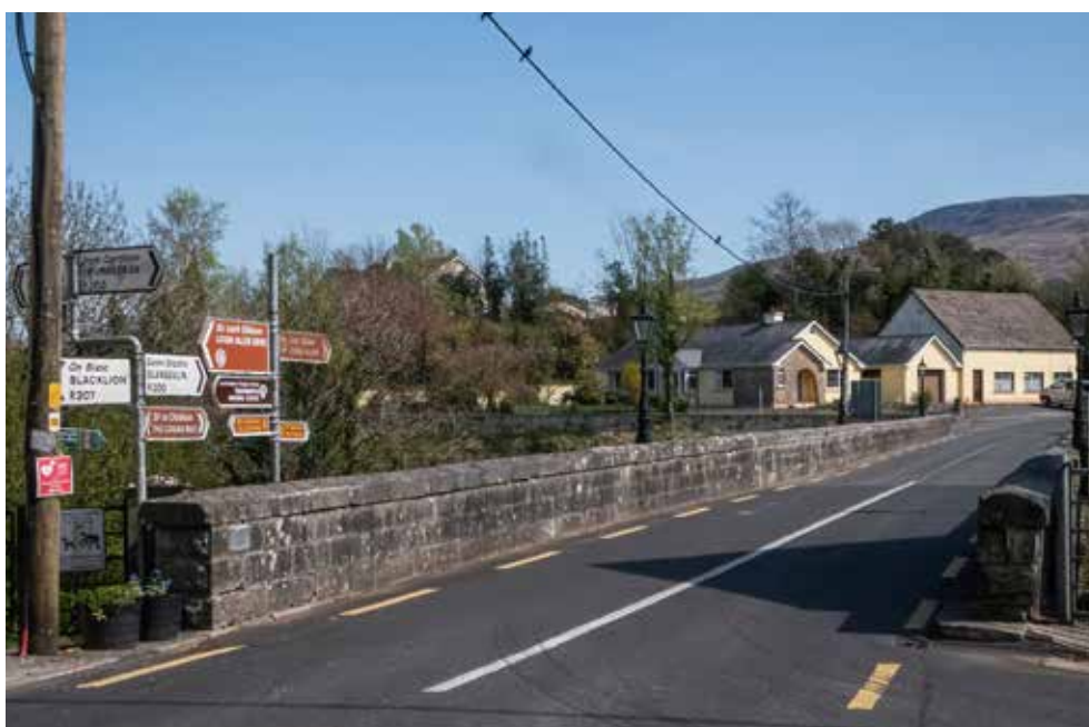
Fig. 11: View of Dowra Bridge.
