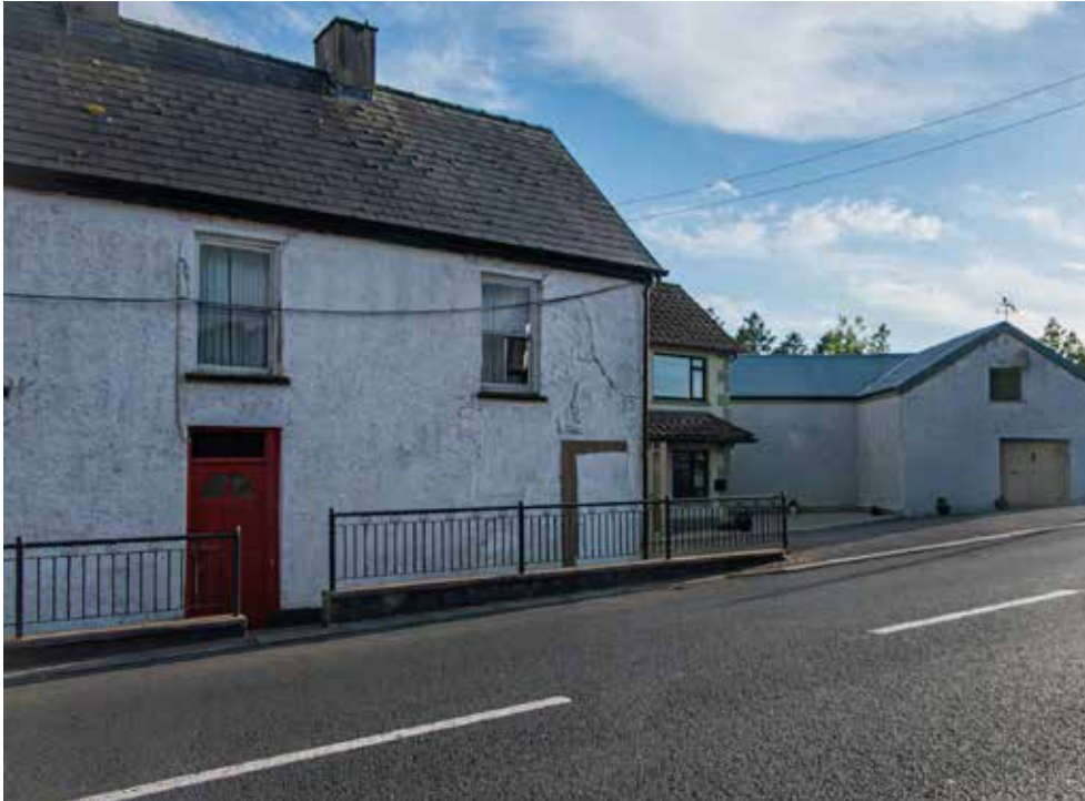
Fig. 13: View of two-storey terrace on the western end of the street and the former mill building.
