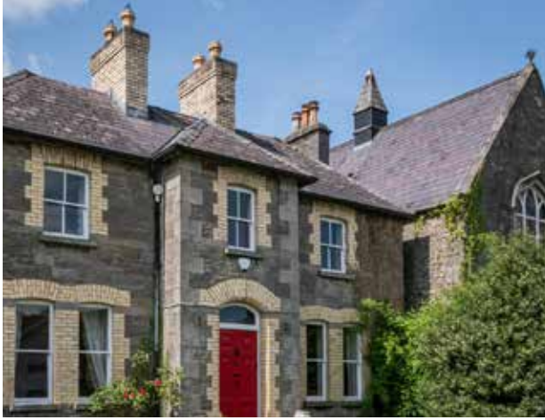
Fig. 14: Historic architectural features including natural slate roofing, and brick chimneystacks.
