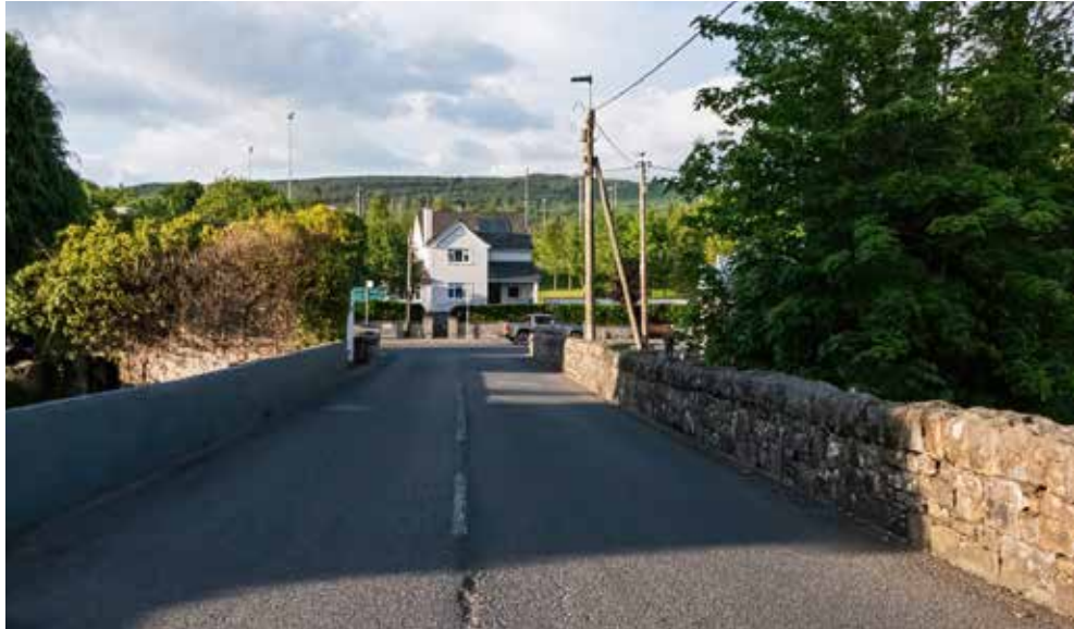
Fig. 11: Road bridge crossing over the River Bawnboy on the southern approach road to Bawnboy.
