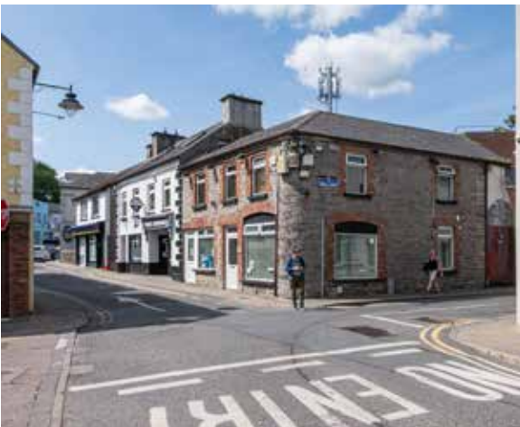
Fig. 13: View of the junction of Bridge Street and Abbey Street.
