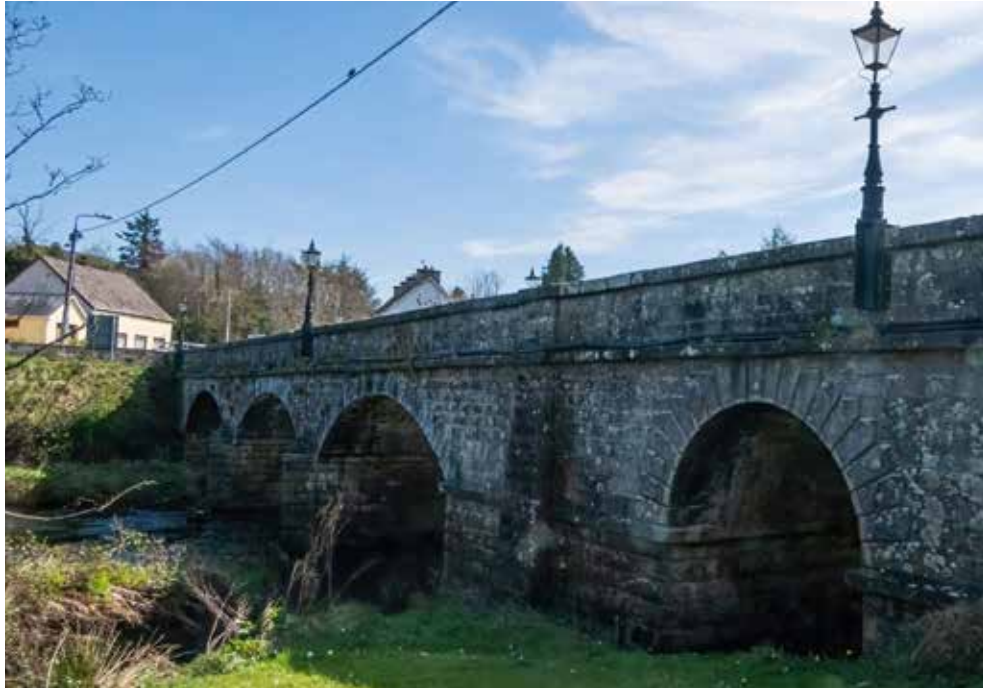
Fig. 12: View of the north face of Dowra Bridge. The architectural detailing and the use of tooled stone makes this an important architectural feature in the village.
