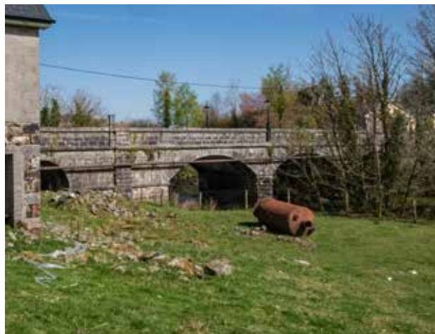
Fig. 14: View of the south face of Dowra Bridge.
