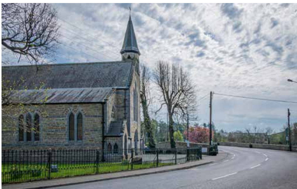
Fig. 13: View of St Aidan's church and road leading towards the bridge.
