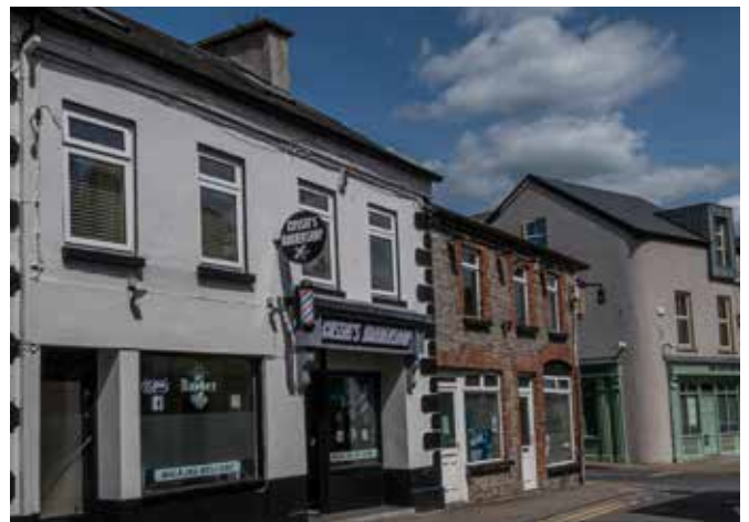
Fig. 23: Shopfront removed from building on Bridge Street.
