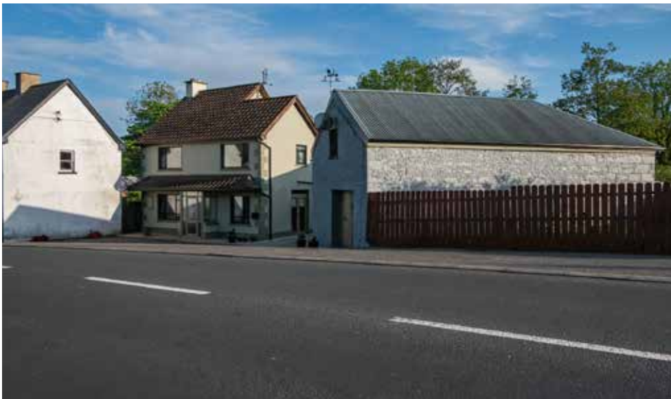
Fig. 14: View of mill building as seen from western end of the street.
