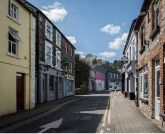
Fig. 17: Mixture of materials and building heights on Bridge Street.
