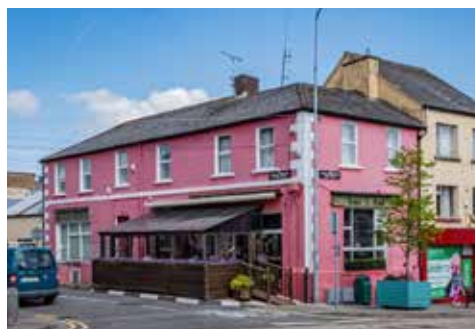
Fig. 17: Building on the corner of Castle St and Butler St.
