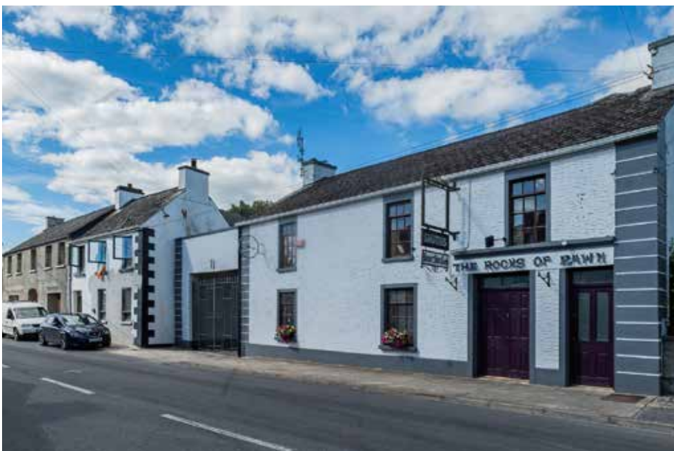
Fig. 10: View of north side of the Main Street. Different roof heights and building lines amongst buildings.
