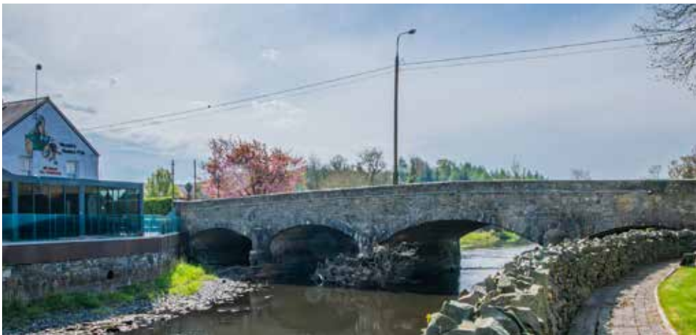
Fig. 14: View of the bridge and neighbouring Derragarra Inn taken from the grounds of St Aidan's church.
