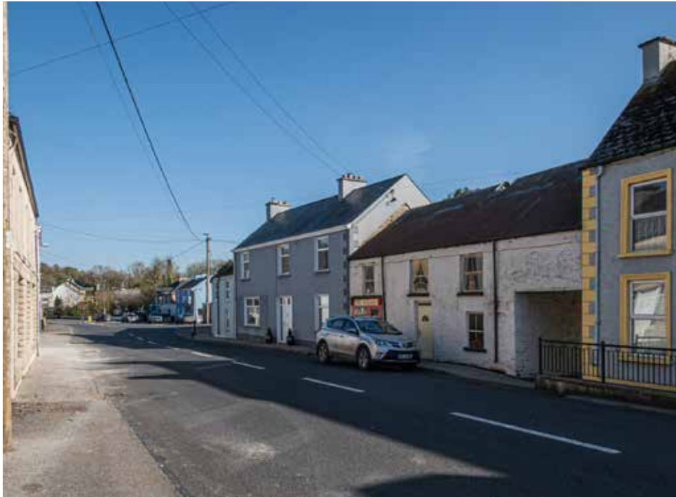
Fig. 15: Pitched roofs and square-headed window openings are common in the village.
