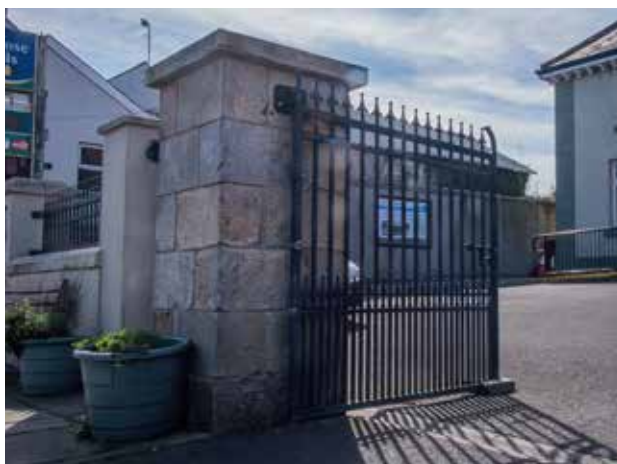
Fig. 17: Entrance piers and railings to the courthouse.
