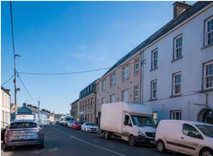
Fig. 11: View of two-storey terrace on the northern side An Bonnán Buí.
