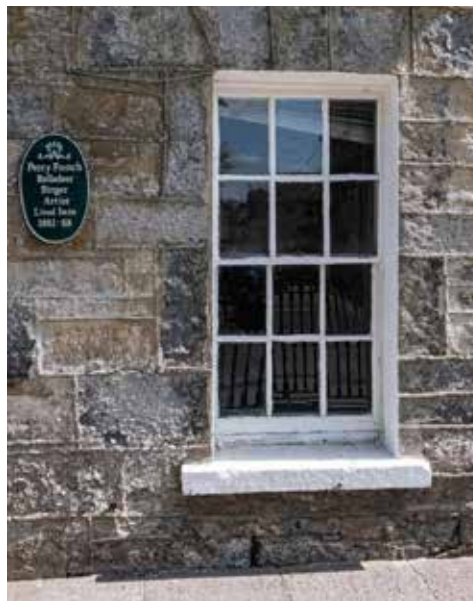
Fig. 15: Original doors and windows on Farnham Street contribute to the historical character of the ACA.
