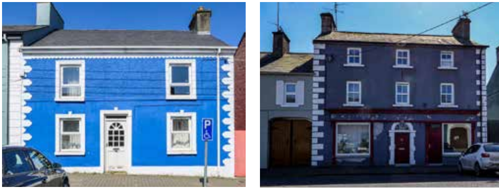
Fig. 7: Example plasterwork finish located within the ACA.
