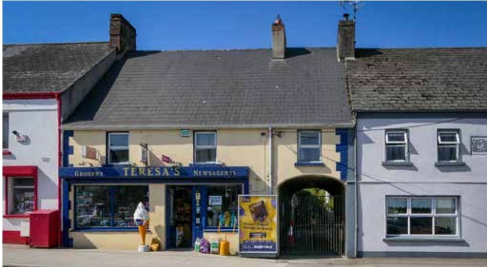
Fig. 23: Typical example of an integrated-carriage arch giving access to a rear site.
