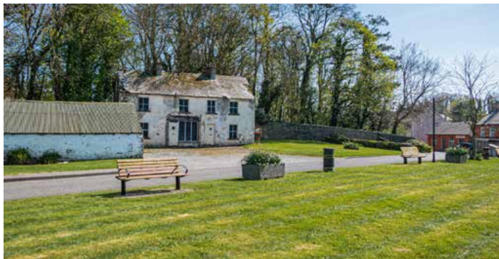
Fig 13: View of the former Constabulary Barracks on the south-western side of the Fair Green Public benches, bins and planters located along southern side of green.
