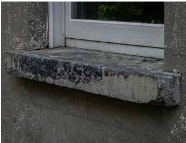
Fig. 33: Tooling marks on stone threshold and windowsill.
