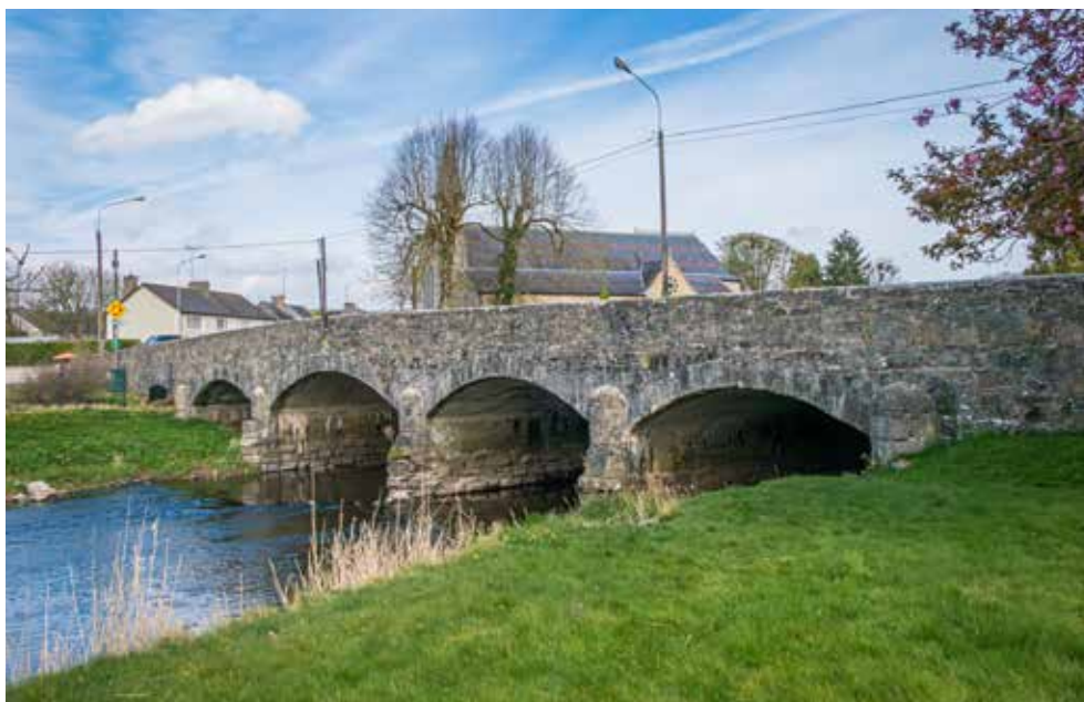
Fig. 12: View of the bridge at the southern end of Butlersbridge village.
