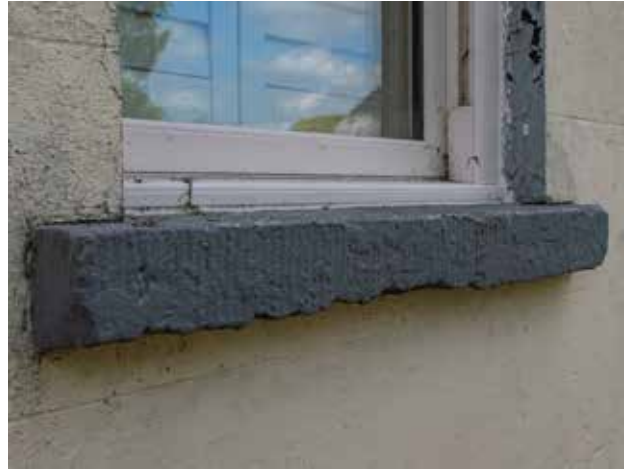
Fig. 32: Detail of tooling on windowsill.
