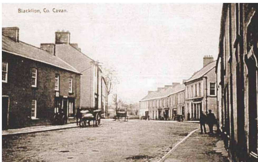
Fig. 6: Blacklion - View westwards up Main St. in the early 1990s. The tall building on the right hand side of the photo with a shopfront and round-headed door opening was demolished and replaced by the Garda Station.
