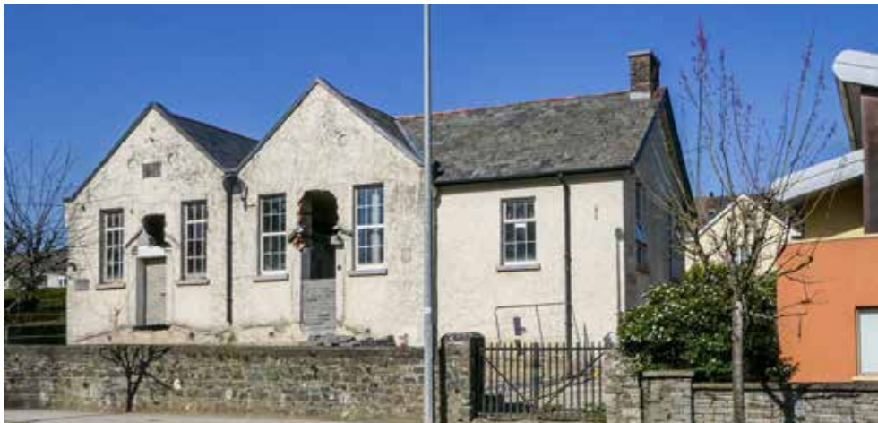
Fig 13: Former National School on Cavan Road.
