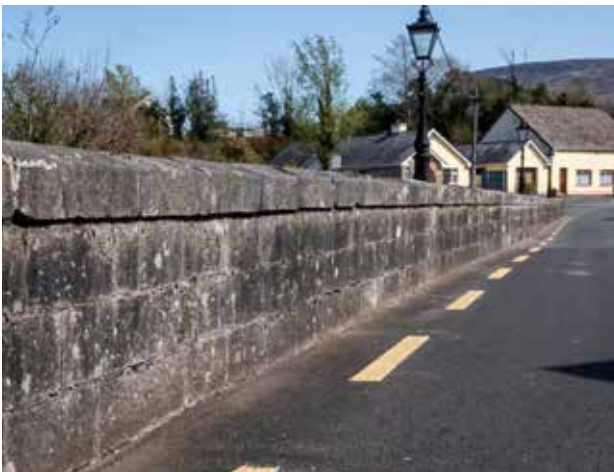
Fig. 13: View of the parapet on Dowra Bridge.
