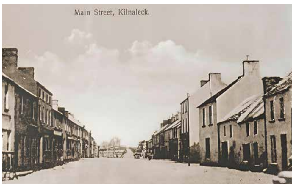
Fig. 8: Historic photograph taken in Kilnaleck Village, date unknown, c.1910 This photo was taken at the southern end of Main Street. Two three-storey buildings face each other on Main Street at the junction in the road. The remaining buildings in Kilnaleck are predominantly two-storey tall.
