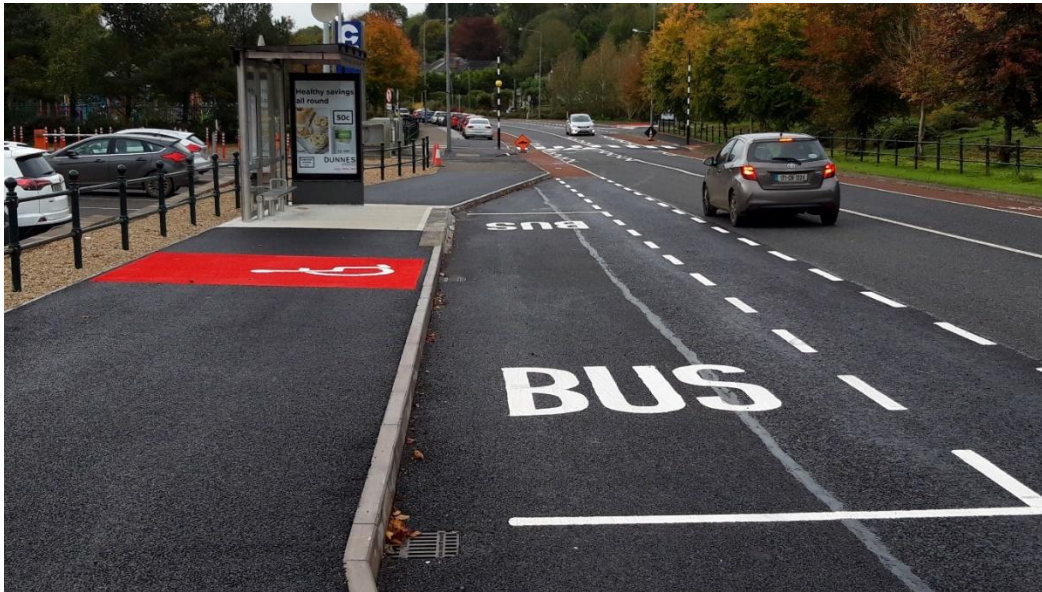
Fig 7.1 New bus bays, cycle path & pedestrian crossing at Cavan Institute of Technology 2019
