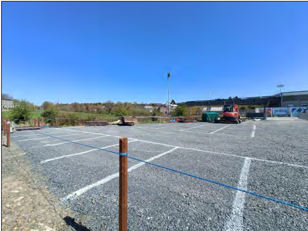
Figure 22. GAA carpark in south area of site
