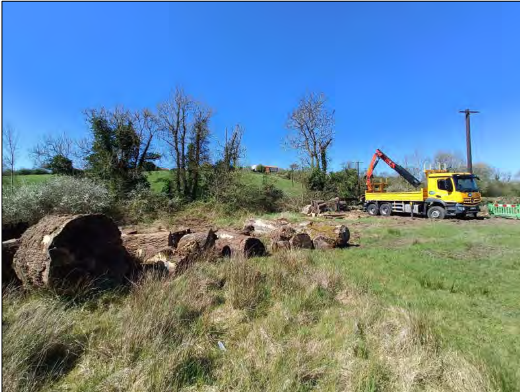
Figure 28. Current on-going works on site
