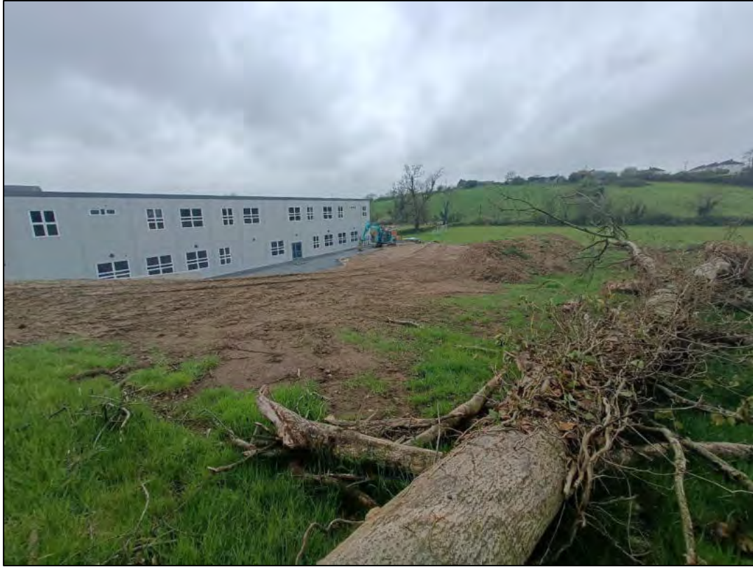
Figure 21. Felled trees from cleared treeline, bare ground and new school building
