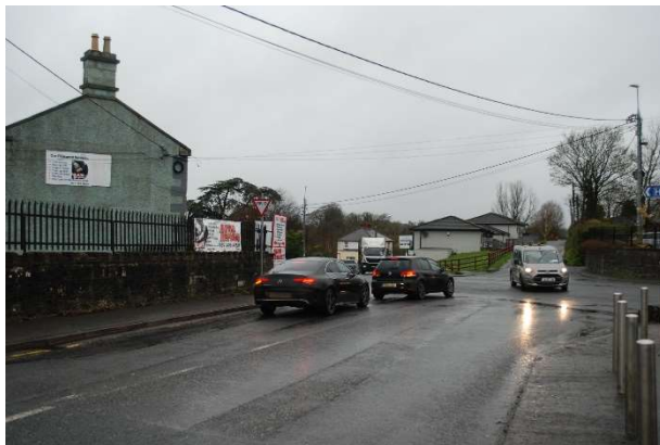
Cavan School to LHS
