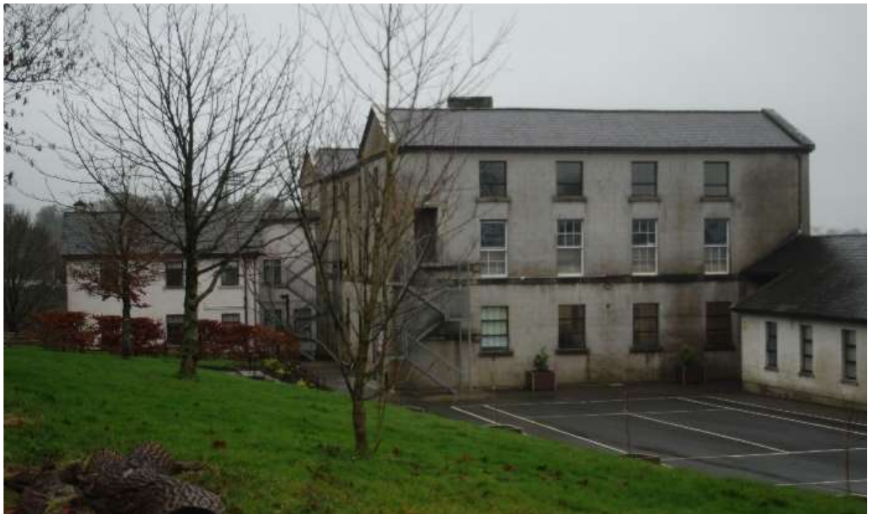
Rear (North) of School buildings unaffected by proposed works
