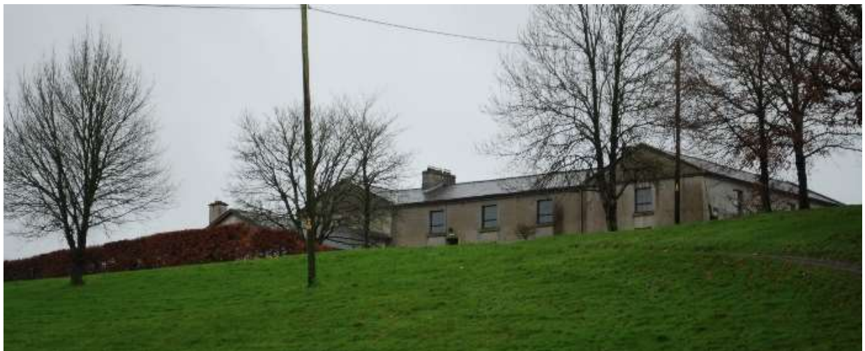
View of School on elevated site
