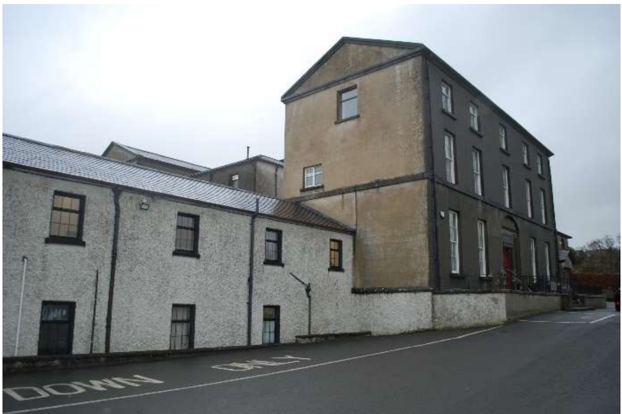
School to RHS (East) and Outbuildings to LHS (West) – Both Protected Structures with separate designations
