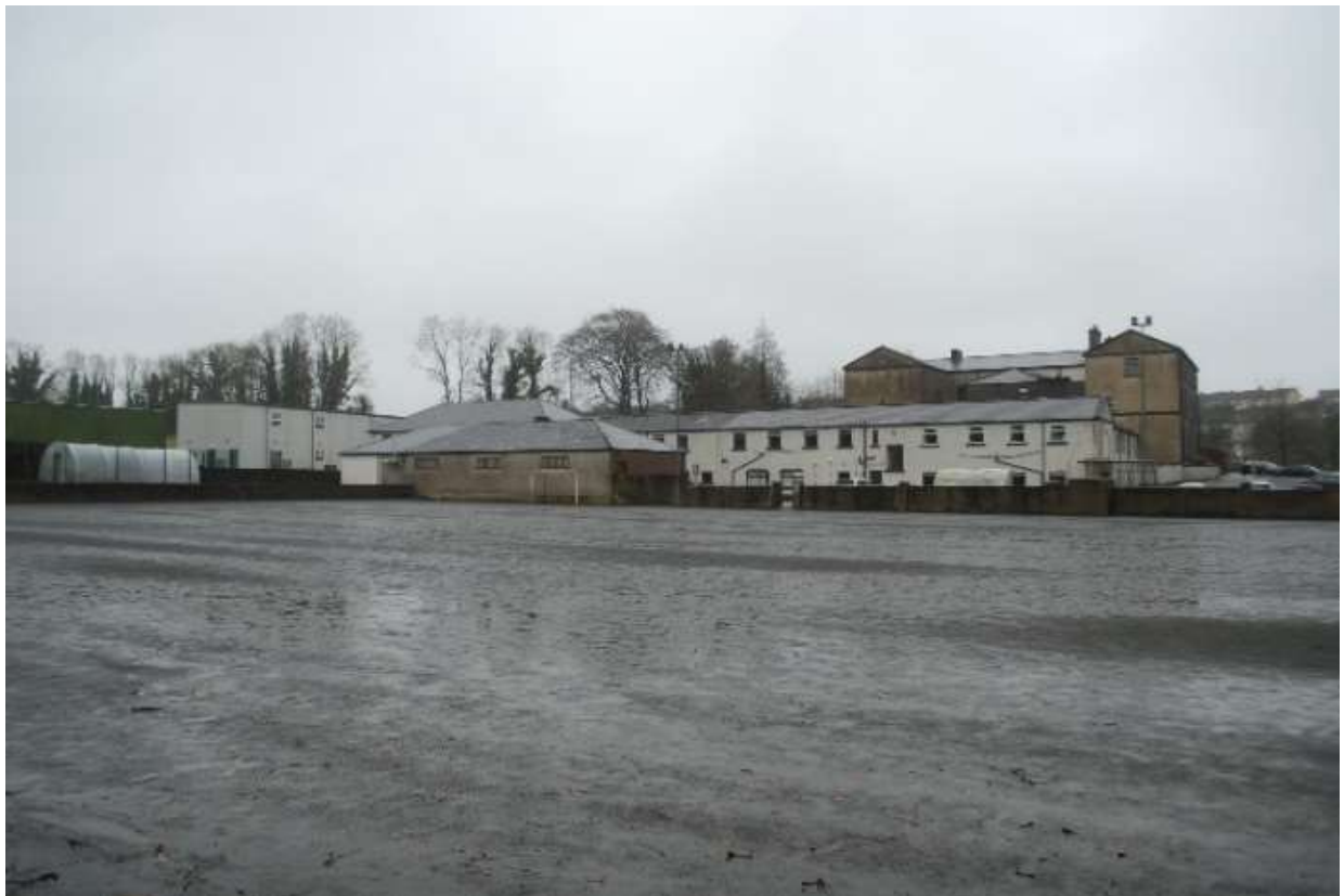
View across all weather pitches to the east towards the school behind outbuildings
