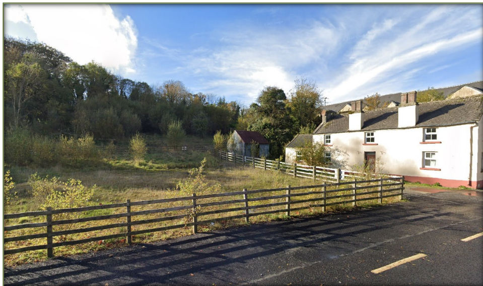
Figure 4b – Google Street View Oct 2022 © Google
