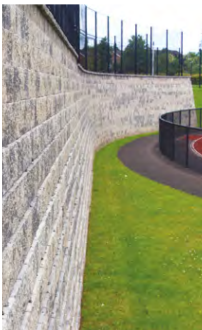
Walling & Retaining Walls
