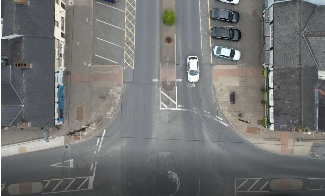
Figure 4 – Pedestrian Crossings on Main Street at Kells Road roundabout
