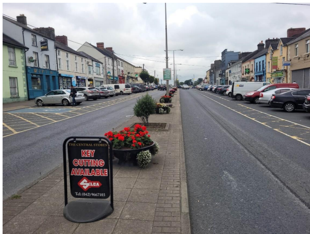
Dual carriageway arrangement with poor median design
