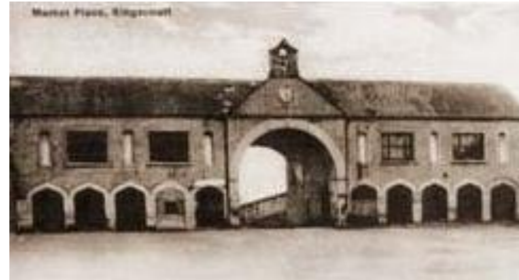
Original market building at western edge of square (demolished)
