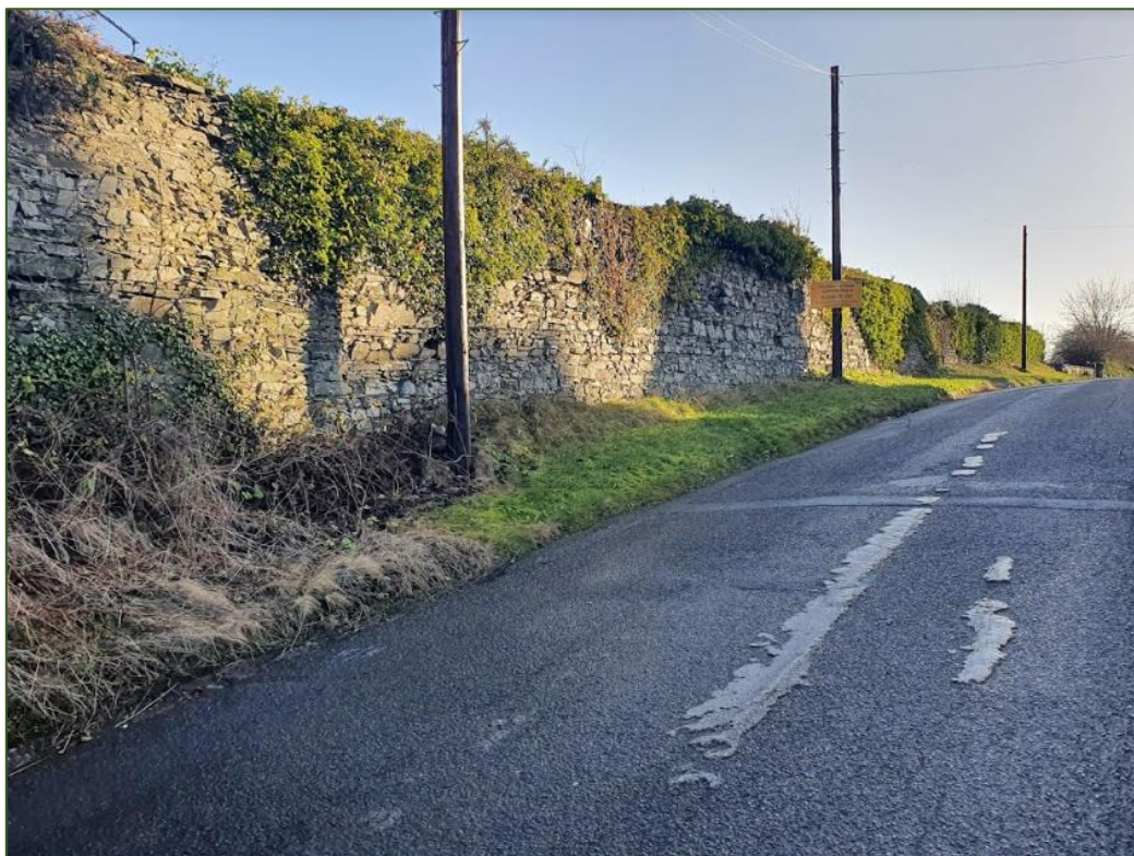
Image 4 Stone wall along St. Mary's Road
