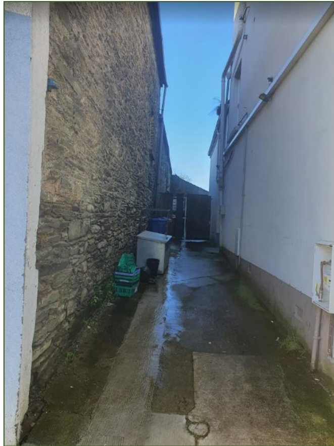
Image 3 Lane to south of Centra showing stone-built gable of building to be demolished.
