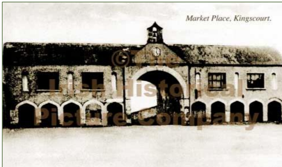
Figure 9 Market House, Kingscourt.
