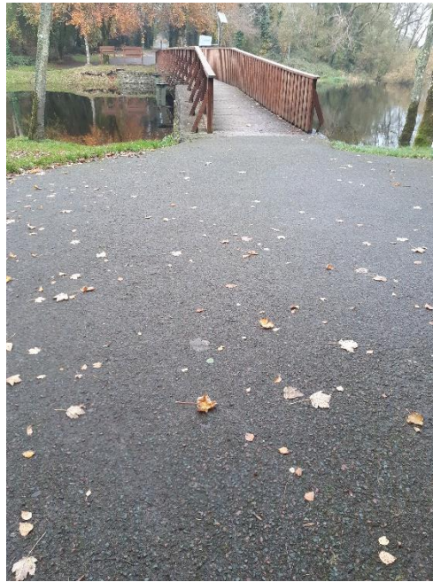
The Eastern End of the Bridge, Looking West
