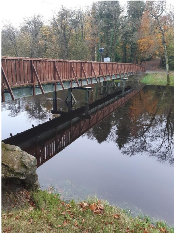
A View of the Bridge from the Western Shore, looking North
