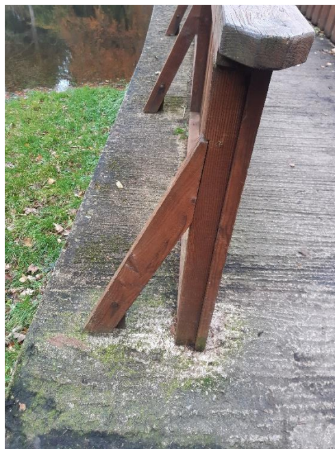
Abutment at the Eastern End
