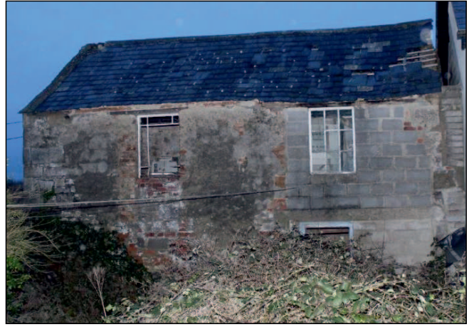
Plate7: Rear of two storey stone structure at rear of PDA
