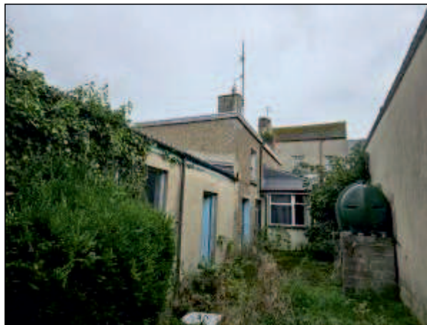
Plate 5: View towards derelict dwelling and apartment building to the rear of Main Street
