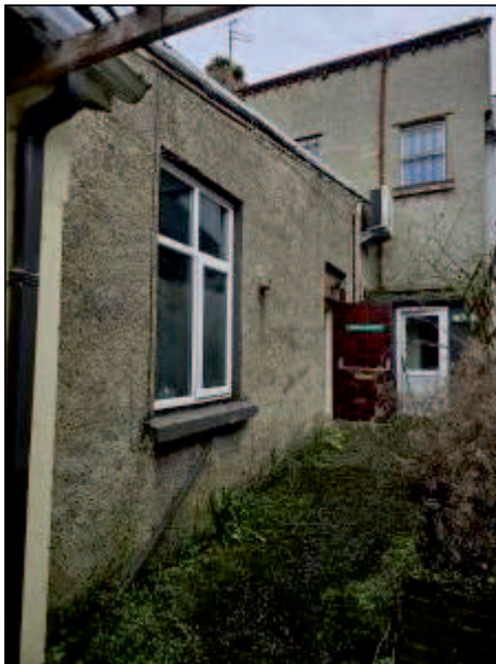
Plate 3: View towards rear elevation of building and single storey rear extension
