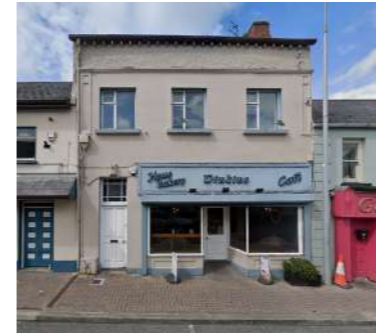
Site Photos - Former Dinkins Building
