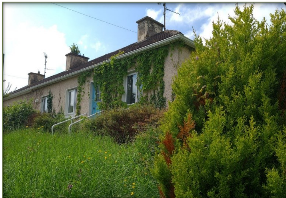
Figure 5c – Existing Derelict House
