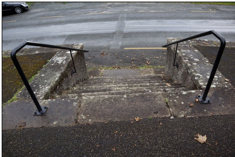
Figure 5: New handrails fitted to steps
