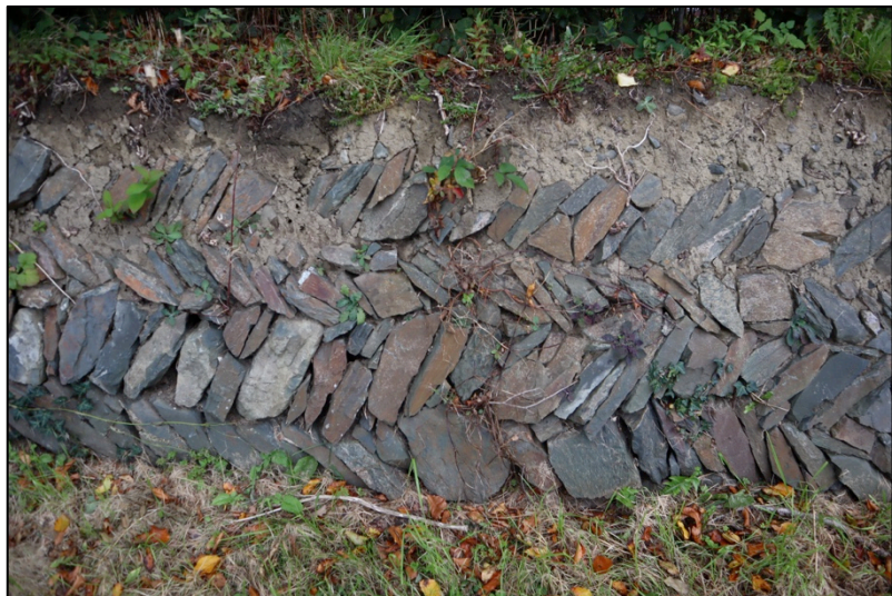
Figure 15: Detail of herringbone wall bounding part of Ballyhaise College land at end of raised path
