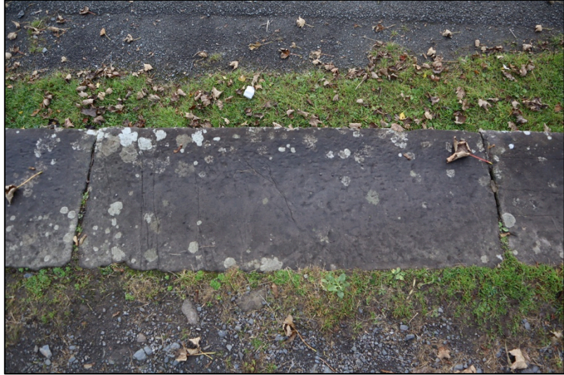
Figure 13: Detail of limestone flat coping stones forming edge of raised path
