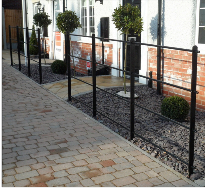
Suitable railing type: Flat-iron posts.
