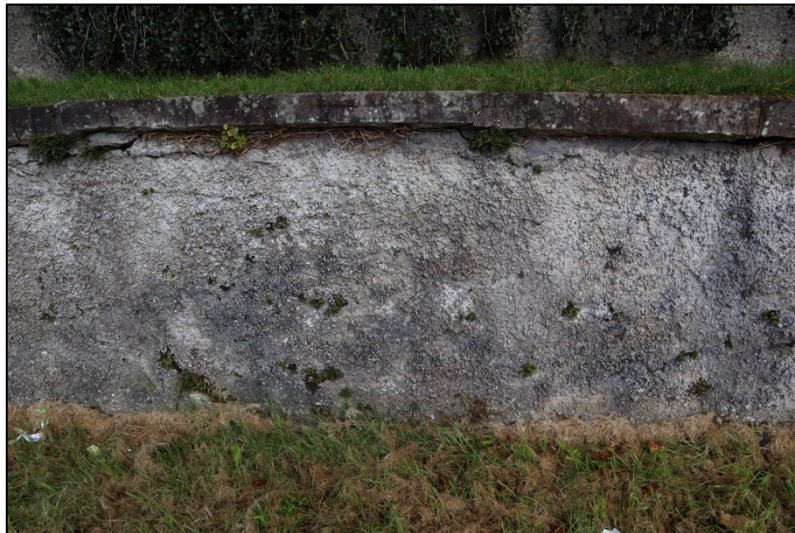
Figure 8: Detail of rendered raised wall with flat copingstones
