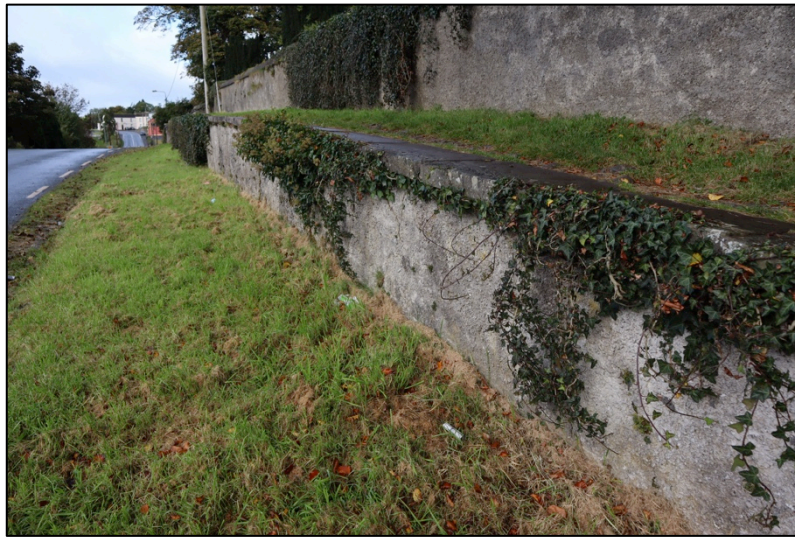
Figure 7: View of retaining wall to east (Ballyhaise College side)
