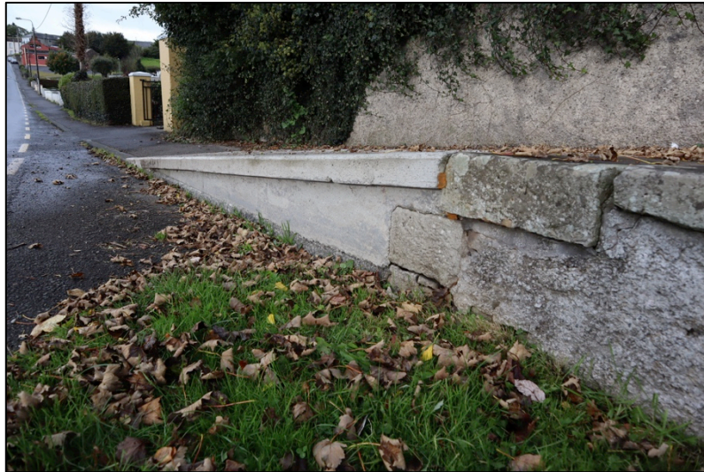
Figure 4: New ramp installed recently at west end of raised path
