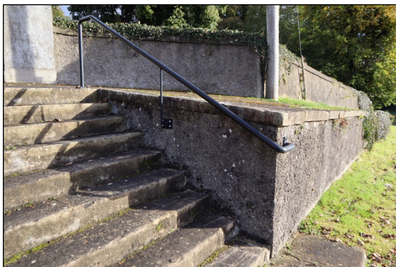
Figure 6: Safety handrail at steps
