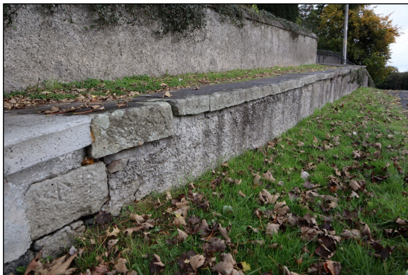
Figure 9: View of retaining wall to west (village side)
