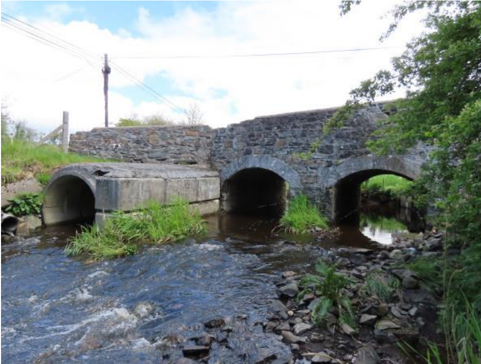
Photo 12 – downstream elevation showing concrete pipe extending beyond other two arches
