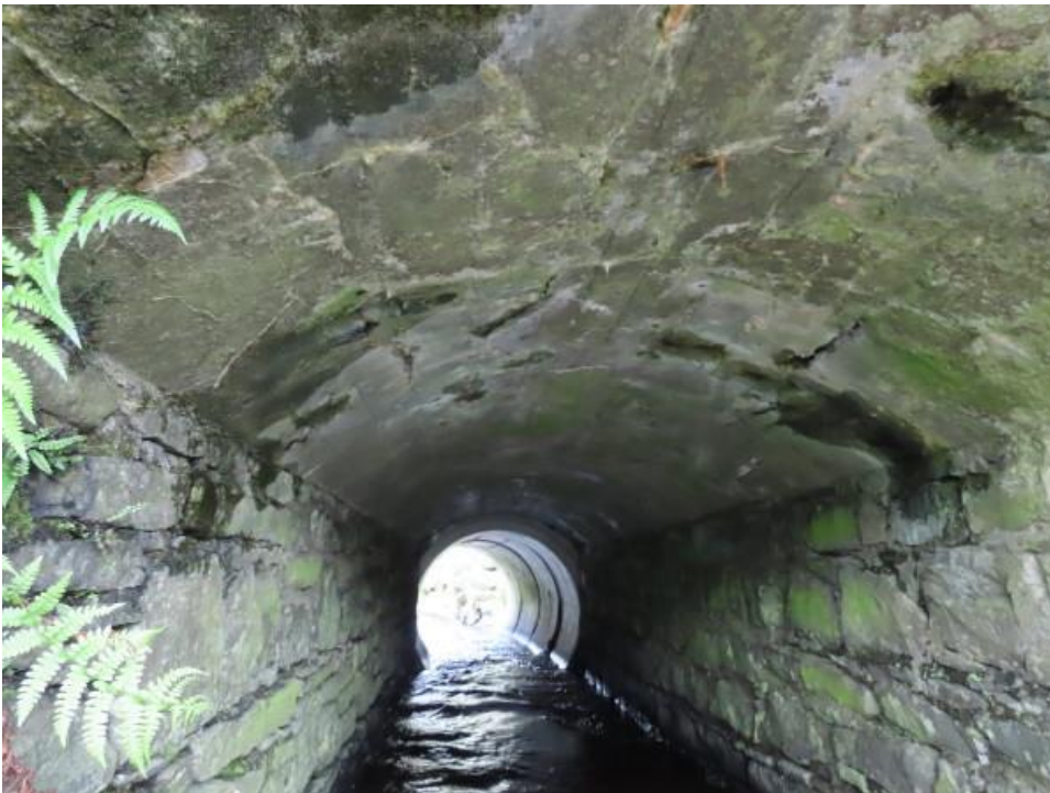
Photo 11 – showing shuttered concrete grout on undersurface of northern arch
