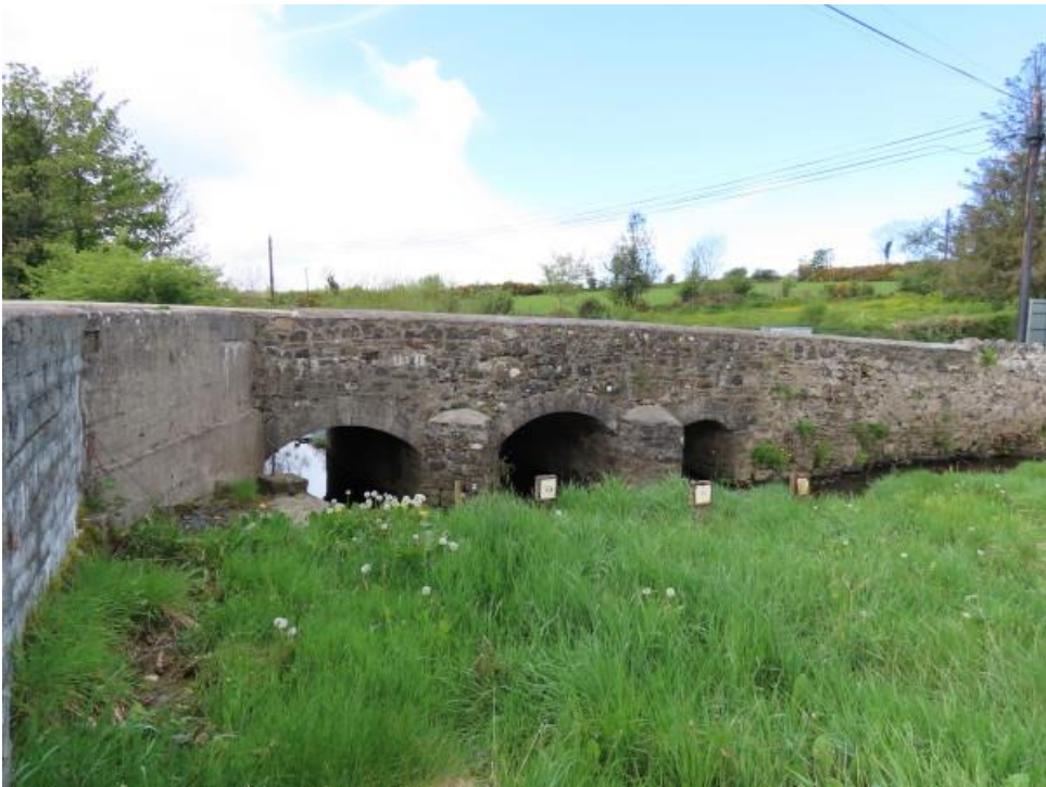
Photo 9 – upstream elevation of existing bridge
