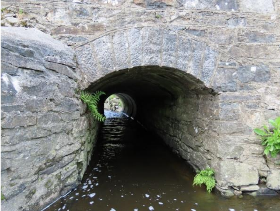
Photo 10 – View under northern arch showing concrete pipe extension at downstream face
