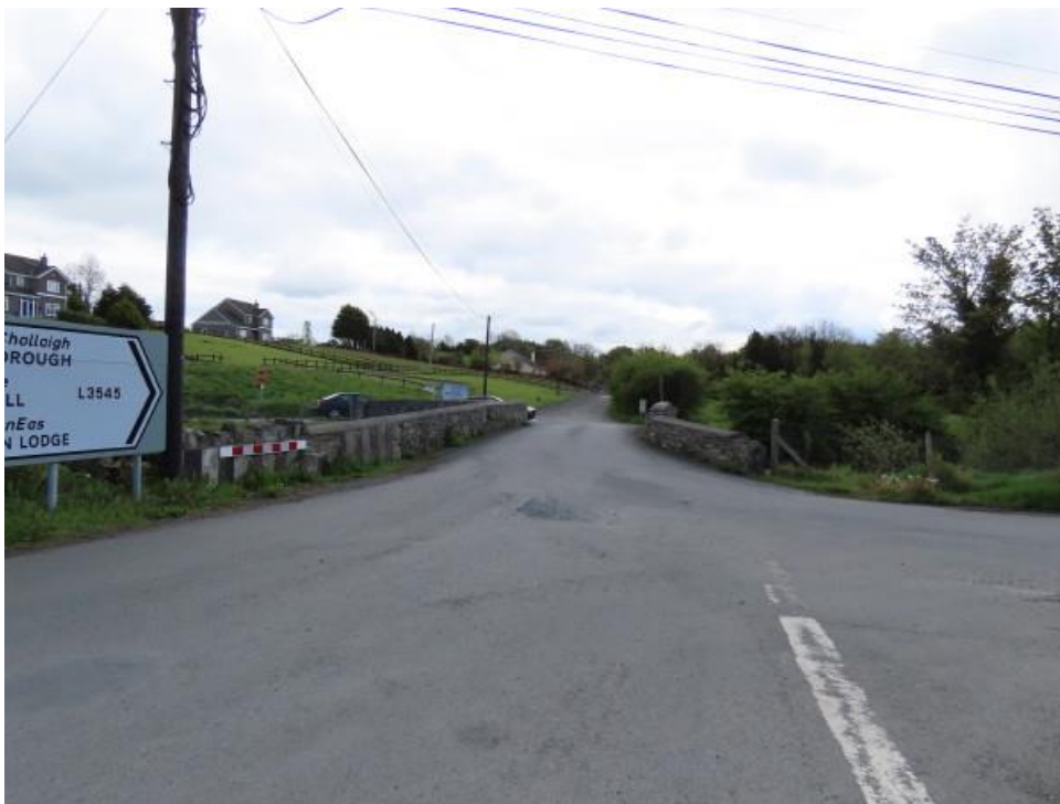
Photo 1 – looking south east across Assan Bridge. The new bridge will be constructed c. 25m upstream of the existing bridge
