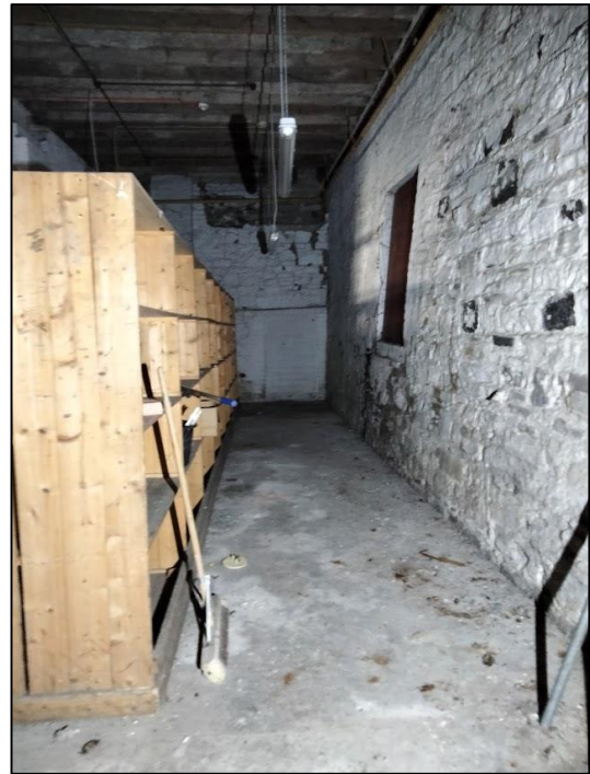
Plate 15. Outer bay of Back Building
