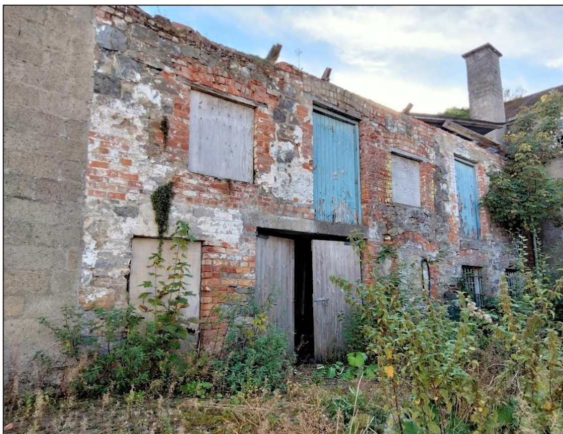
Plate 18. Front of Left Annex. Phot facing south-west
