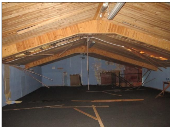
Plate 3. First floor with timber cladding
