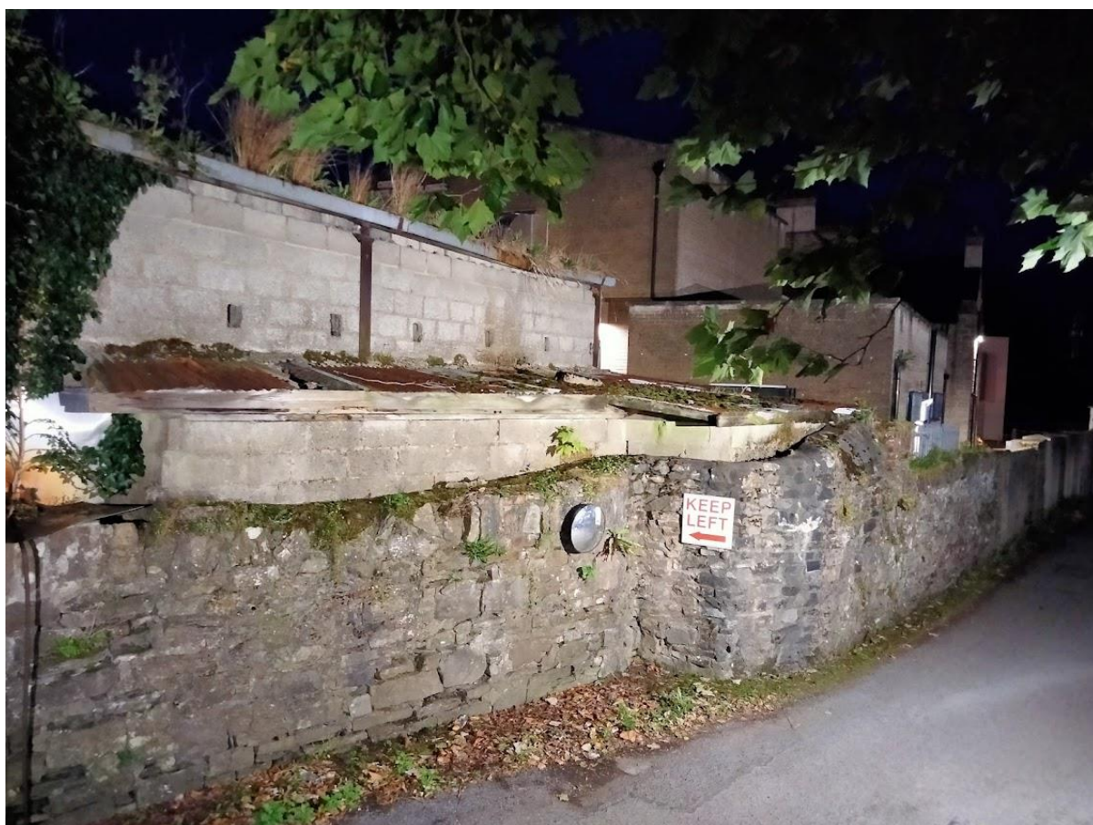
Plate 5. McIntyre's east side is subject to serious light pollution from brightly lit access lane (An Post) which greatly reduces suitability for bats roosting. These lights overspill into the adjacent Abbeyland Park and negatively impact the foraging potential for bats. Photo facing north-west
