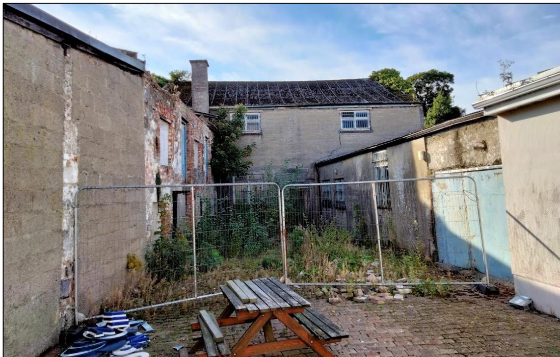
Plate 12. Back Building (centre) with left annex (left) and right annex (right)
