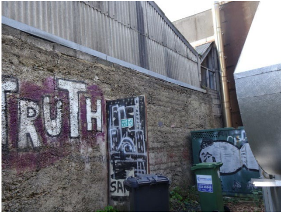
Asbestos Cement (AC) Cladding to the rear Wall
