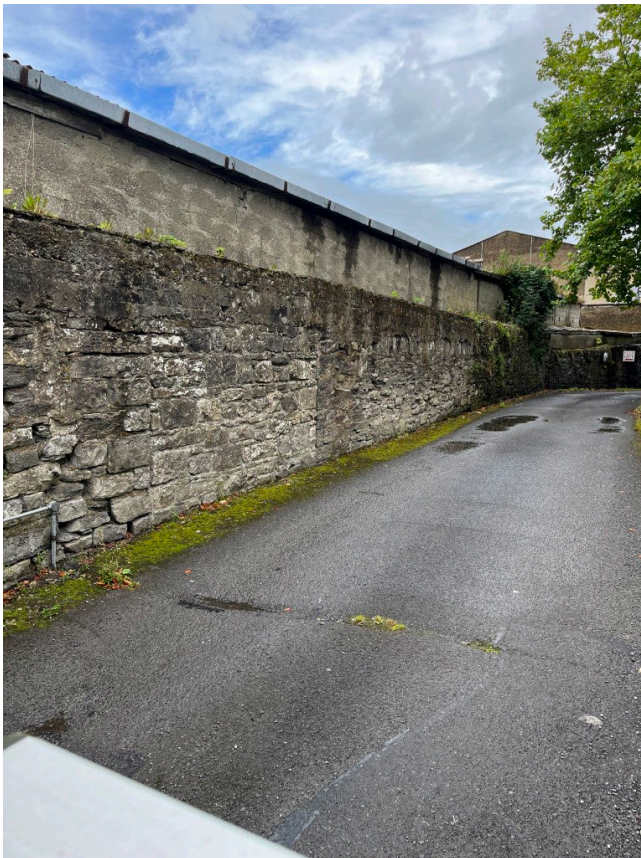
Side wall built inside Stone wall at Right of way
