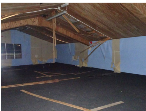
Portalised roof Structure over Mezzanine
