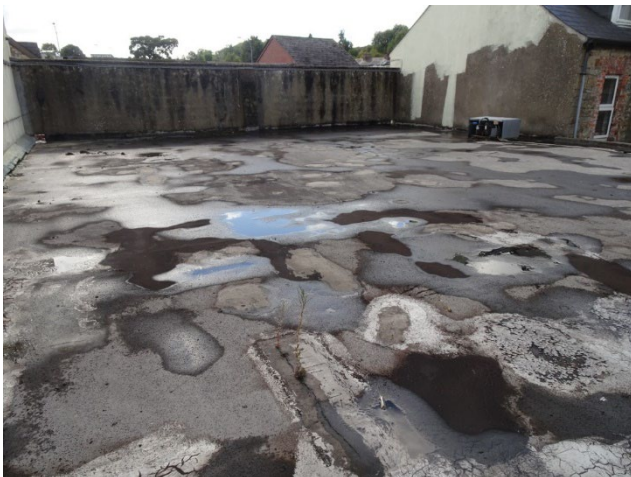
Flat Roof Over Single Storey Area
