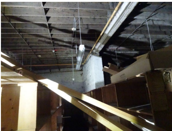
First Floor Joists Supported by Steel Beal on Blockwork Pier A
