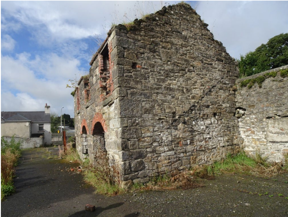
Eastern Elevation Strong Stone Detailing on the Corner
