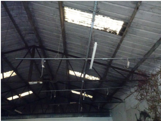
Roof Truss and Asbestos Cement (AC) Roofing
