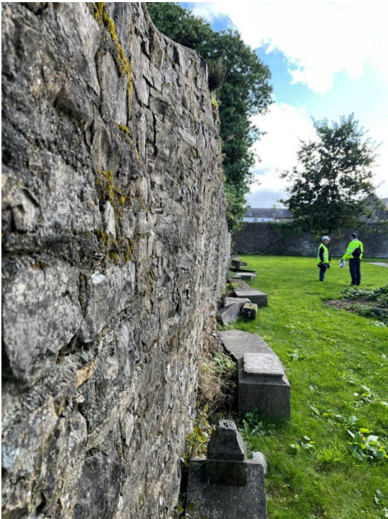
Graveyard Side of Eastern Wall
