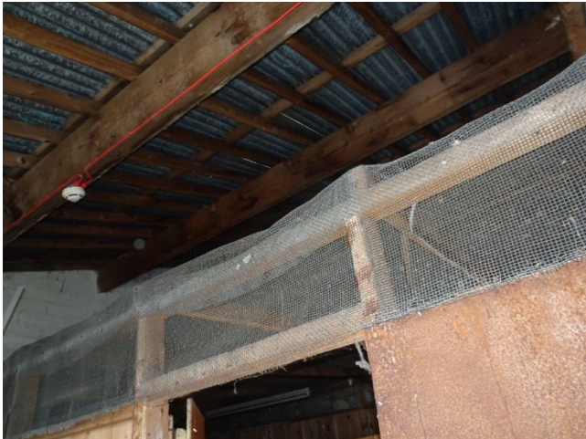
Timber Purlins Support Roof, D
