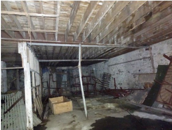
Clear Spanning Steel Beam Supporting Floor Joists B
