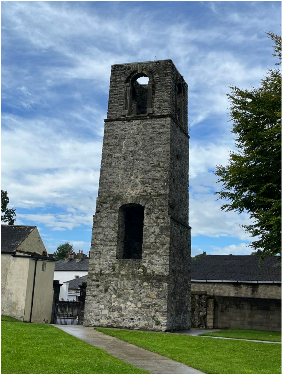
The Existing Tower observed to be in reasonable structural condition
