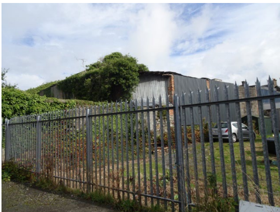
External View Wall Cladding Panels B
