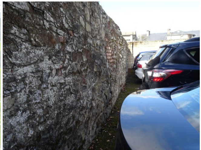
Opposite Side of This wall in the bank Car Park
