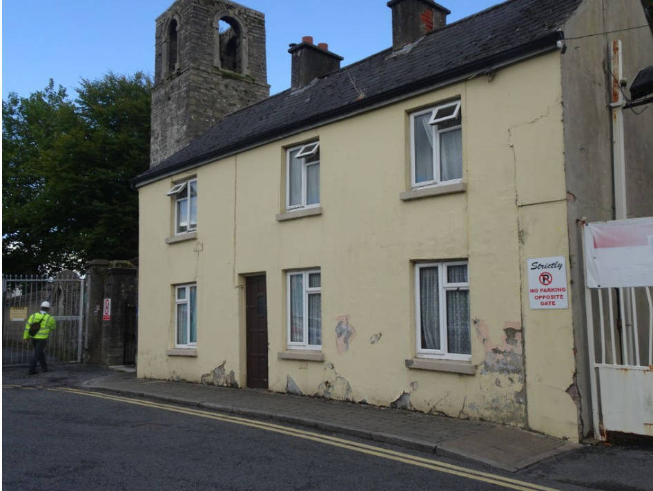
Front Elevation is in Good Condition
