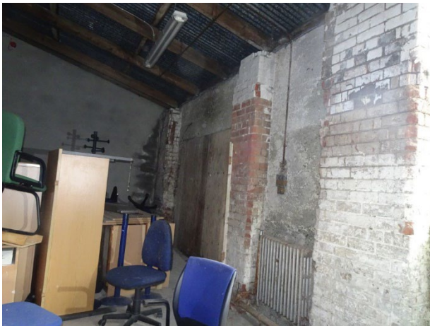
Rafters Support Roof in this area, D
