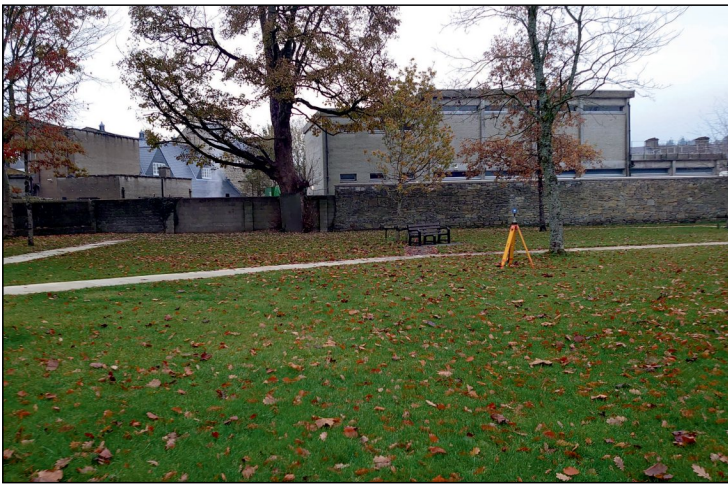
Plate 6: North boundary wall of public space
