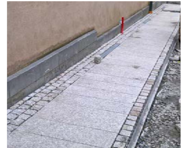
Use of large slabs to provide level, accessible pavements. Setts used to delineate road edge and building line.
