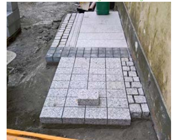
Use of blister paving at uncontrolled crossings, & tactile guidance strip
