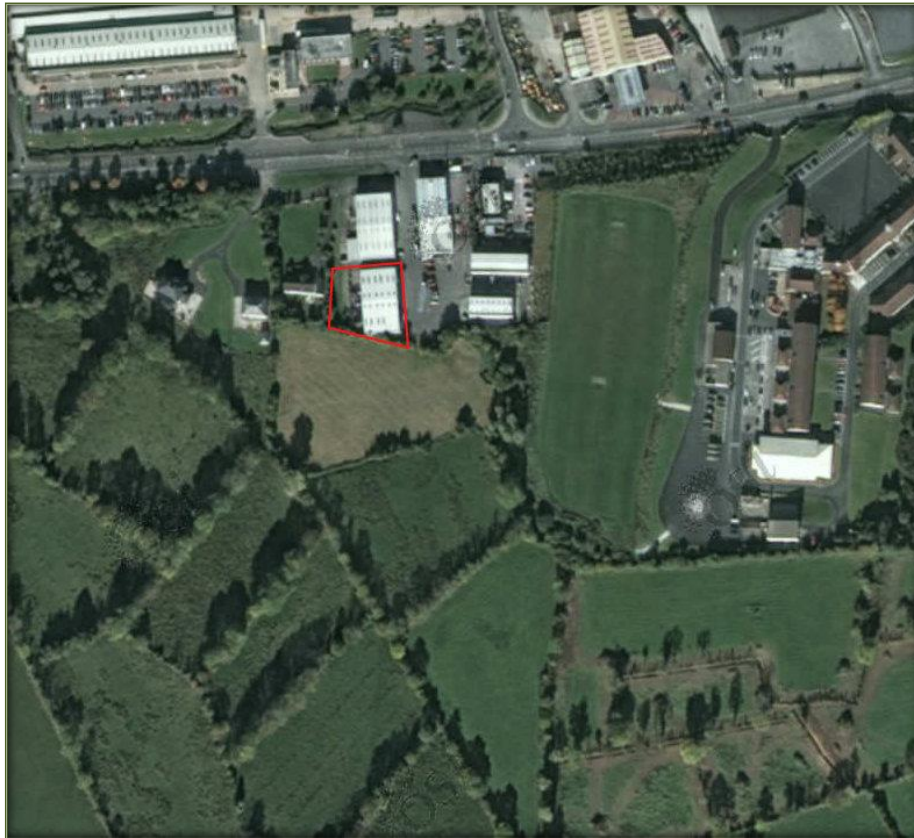
Figure 4 – Aerial Photo of the Site and its Surrounding Habitats
