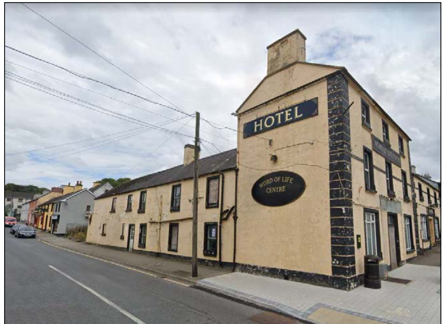
Plate 2: View of former Percy French building and 2 storey adjoining building fronting on to Stradone Street
