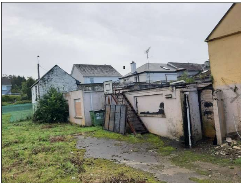
Plate 2: View of modern flat roof extension to rear of development site
