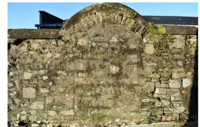
[fig38] 4: Boundary Wall with blockwork infill of archway opposite tower.
