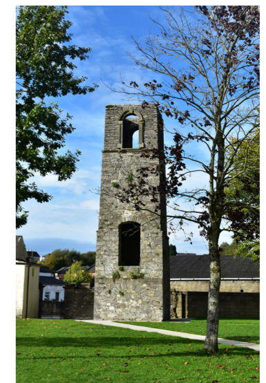
Overall view of tower, looking west.
