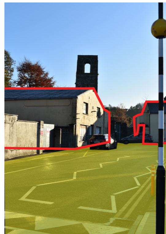
[fig119] Looking from Farnham Street up Abbey Street towards the tower Yellow fill shows extent of public realm improvements
