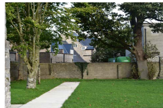
[fig36] 2: Boundary wall with blockwork infill.
