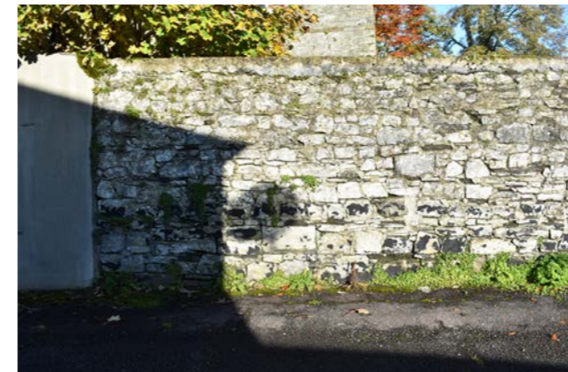
[fig35] 1: Boundary wall opposite former An Post sorting office.
