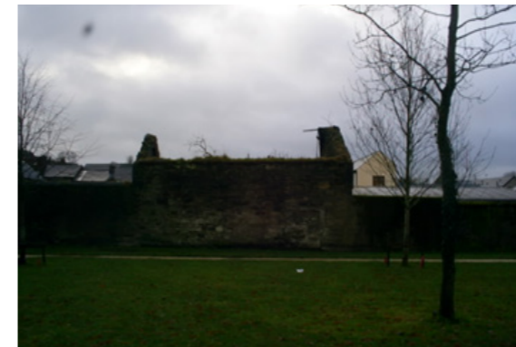
[fig170] Derelict stone buildings such as this would be unlikely to contain bat roosts but would contain potential nesting habitat.
