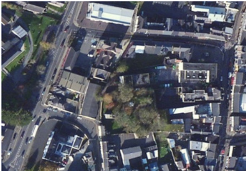
Fig 2: Aerial View of site indicating shadowing. [fig166] A qualitative assessment suggests that the site meets the BRE recommendations referred to elsewhere in this section.
