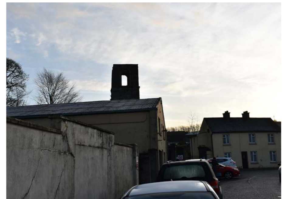
[fig62] Abbey Street with view of McIntyre's & abbey tower, January 2020.
