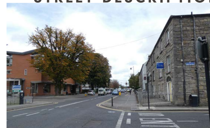
[fig85] The New Library building on Farnham Street. source: dhb architects/Cooney Architects
