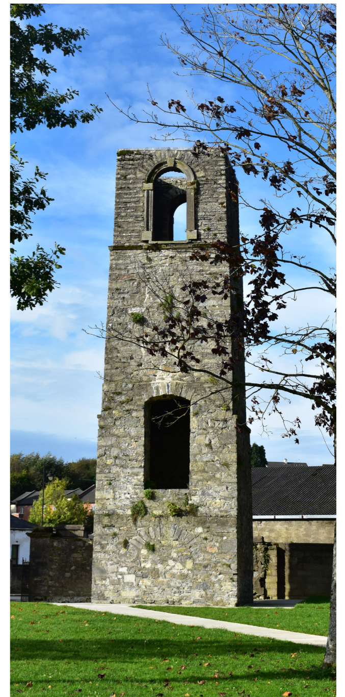
[fig26] View of Tower, looking west.
