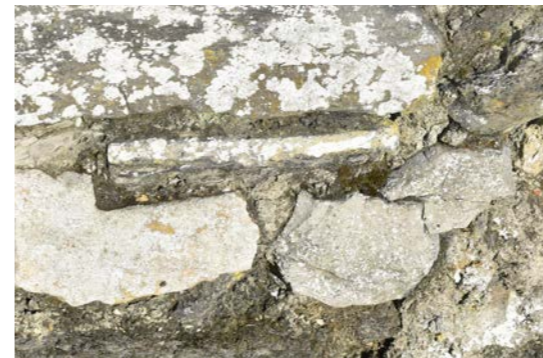
[fig31] 1: Dressed stone visible in boundary wall
