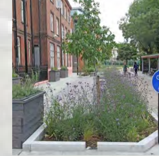
Hard surfaces draining in to soft areas in streets and handstandings – reducing flooding and reproducing natural surface water drainage systems. Soft areas used for mixed native and ornamental planting enhancing ornament and biodiversity.
