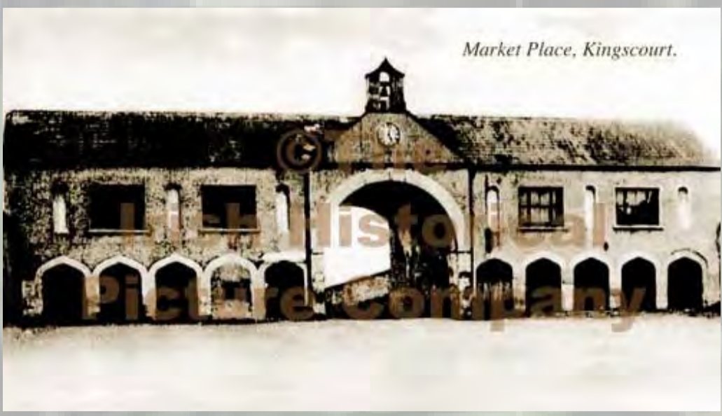
Market Square and its former arched market building
