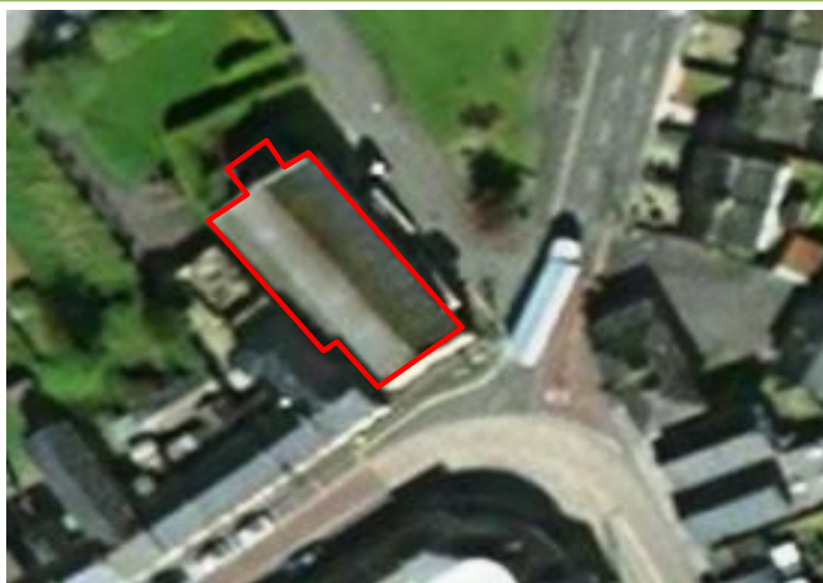
Location of fire damaged Erne Palais Ballroom
