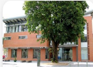
Johnston Central Library Cavan Town
