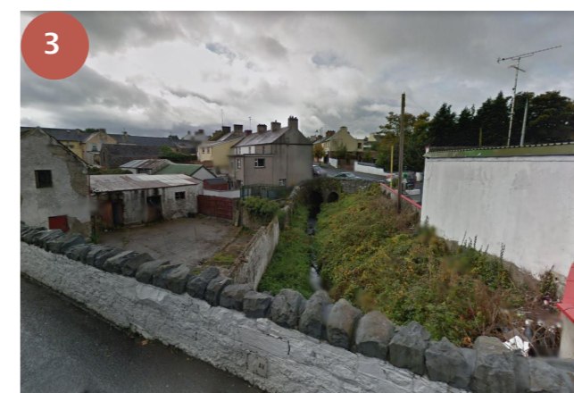
Poorly integrated waterways
