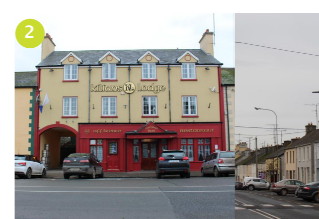
Freshly repainted facade and newly introduced crossing point
