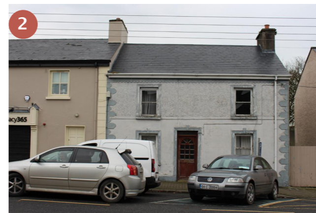
Abandoned premises on the Main Street and chaotic car parking
