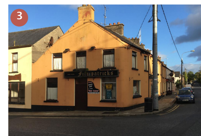
Some buildings are in need of refreshment throughout the village
