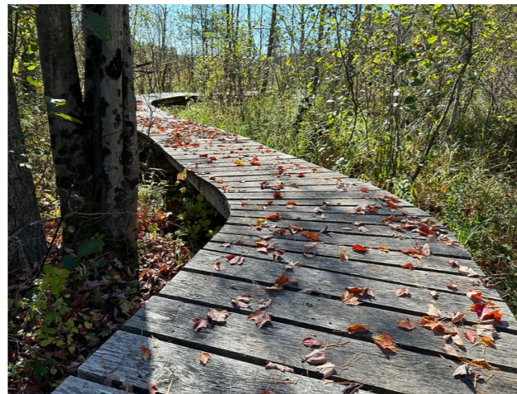
Fig 45 Low impact wetland bridging / walkway (www.ingersolllandcare.com)
