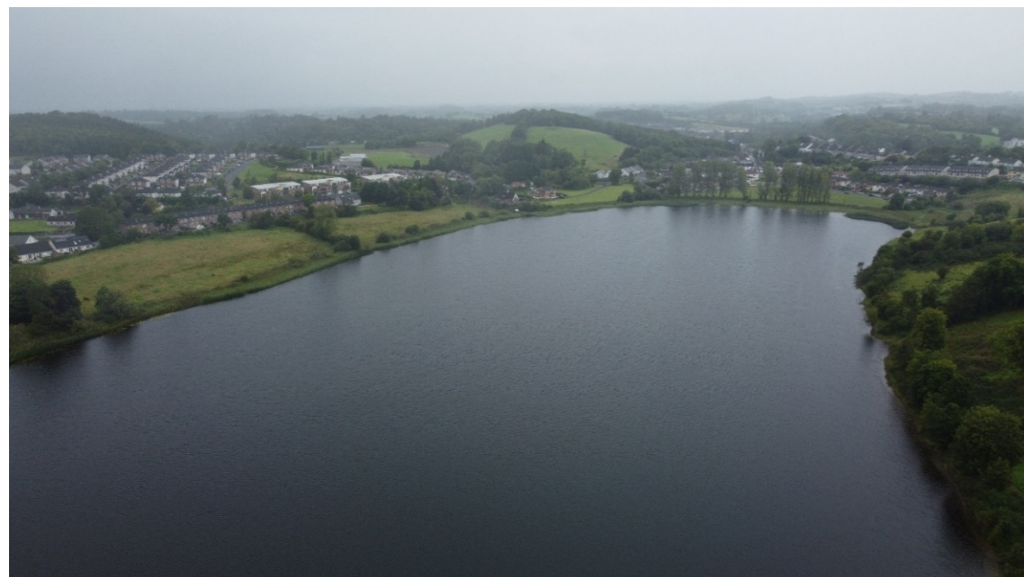
Fig. 10 View north from the southern-most part of the lake – note the contrasting characteristics of the eastern and western banks (from drone survey 28 August 2024).
