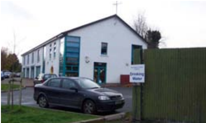
Temporary Public Water Tap – Emyvale Village
