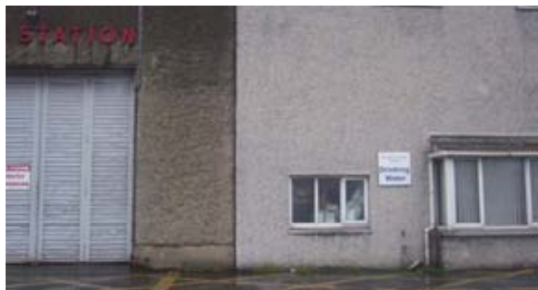
Temporary Public Water Tap – Monaghan Town Fire Station
